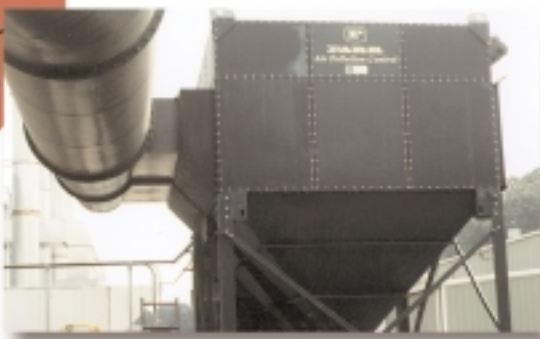
High entry inlet creates a cross flow through the filters. Eliminates upward "can" velocities associated with traditional hopper inlets.
