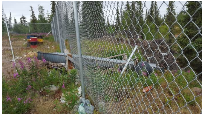
Figure 17.1 - Sewage Truck Discharge Culvert
