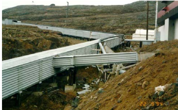
Figure 3.7 - Old Box Utilidor in Iqaluit
