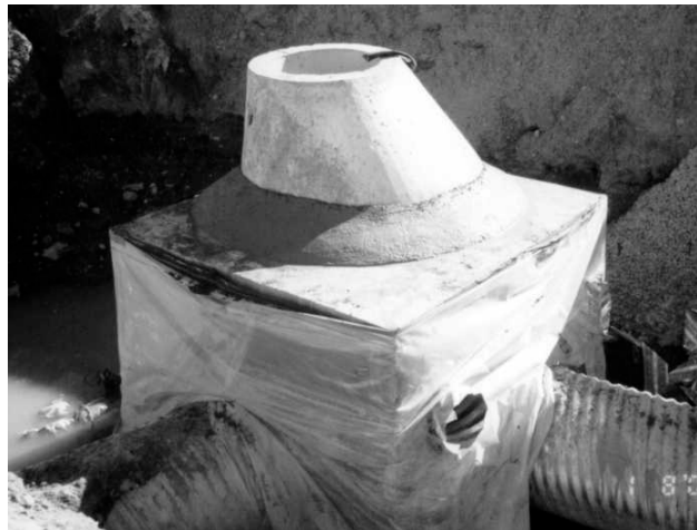
Figure 5.3 - Cast-in-Place Storm Sewer Vault
