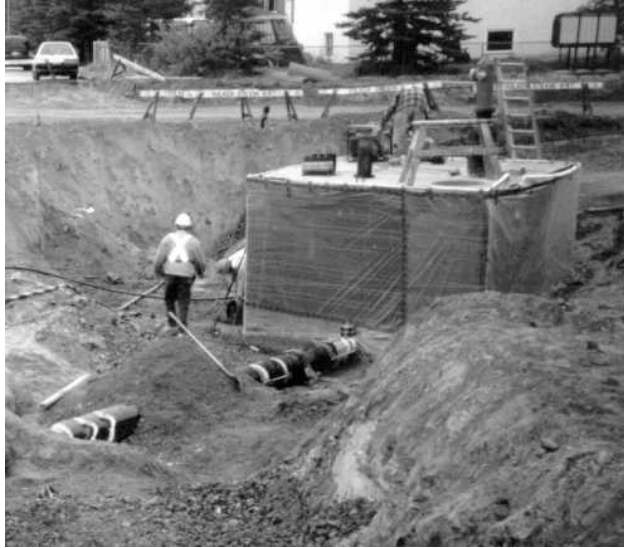
Figure 5.4 - Cast-in-Place Hydrant Vault
