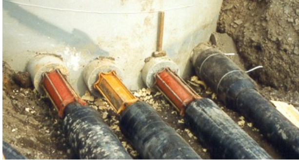
Figure 3.12 - Couplers on HDPE Pipe
