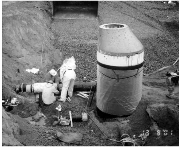
Figure 5.2 - Pre-cast Sanitary Manhole c/w Cone Top and Polyethylene Wrap
