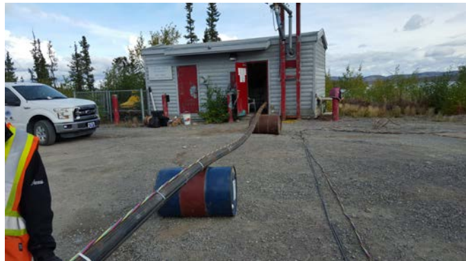
Figure 13.2 – Intake Pipe Supported by Barrels During Pump Pull
