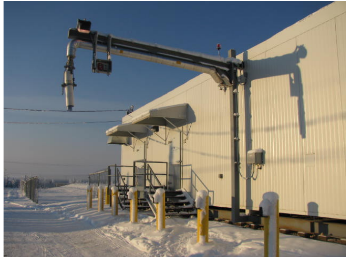
Figure 13.1 – Typical Water Treatment Plant Building
