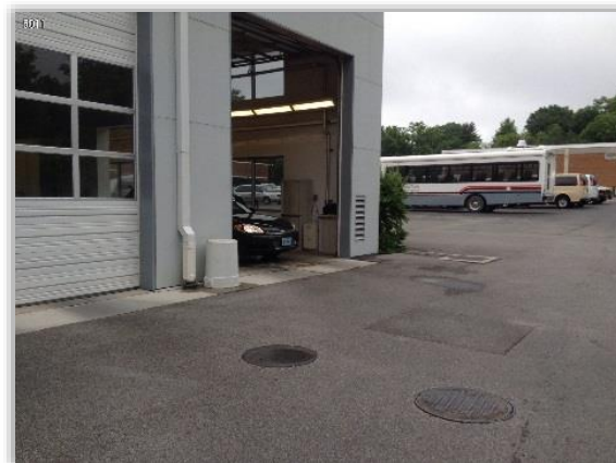
Photo 2: Indoor Wash Bay.
