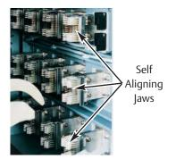
**Fig. 7:** Bypass-Isolation Transfer Switch self aligning power jaws.
