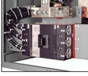
**Fig. 10:** Ground and neutral disconnect links
