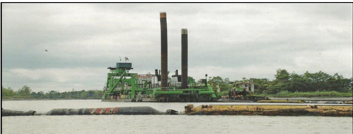
Figure 4.9 Dredges in Operation at Bige
