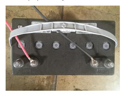
If your battery has sufficient charge (11.5 volts or more), you should now see a single green flash repeating on the charge controller's LED display. This means the controller has power (controllers are powered by the battery, not the panels).
