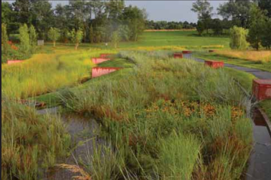
Bioretention Pond at North Carolina Museum of Art, Raleigh, NC Photo credit: Stephen H. Blake, P.E., Artifex Environmental Design, Inc.
