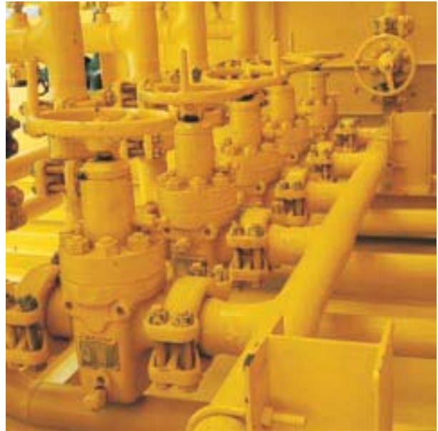
The use of Grayloc connectors, on a Centex Oil and Gas, Inc. platform in the Gulf of Mexico, saved 15" of horizontal space on the separator manifold of this skid-mounted production unit, and reduced the total topside platform weight by more than 11 tons.
