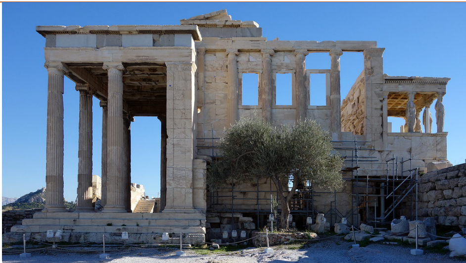
West Façade with partly engaged columns
