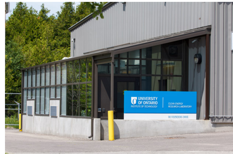
Clean Energy Research Laboratory at the University of Ontario Institute of Technology.
