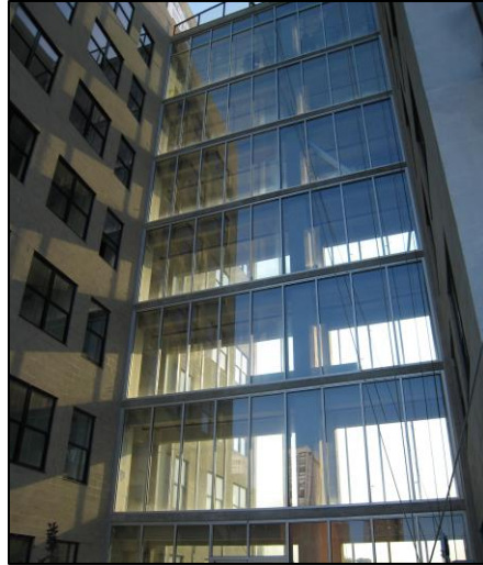
Figure 3.2.2.5.1: Example of fully glazed passageway
