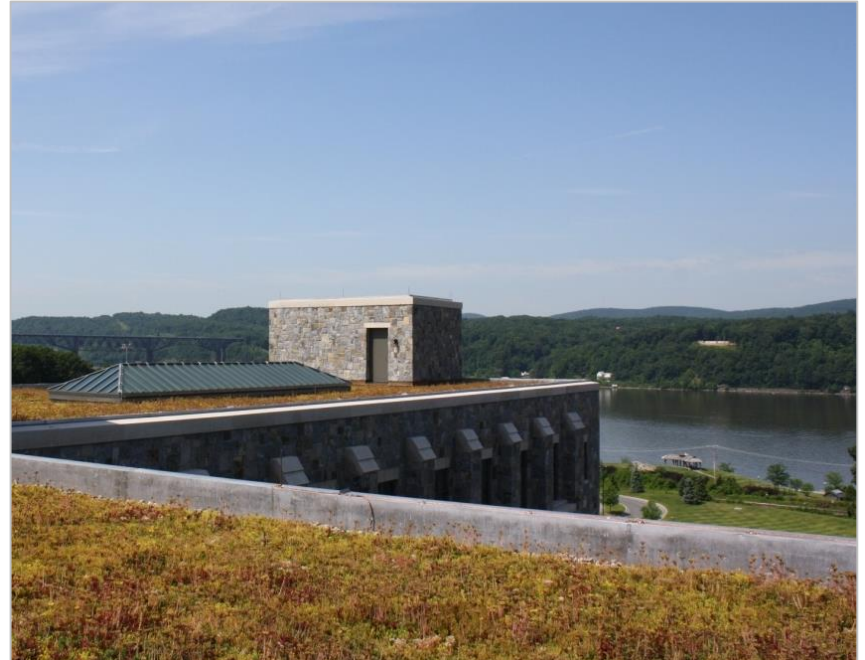
Green Roof at Marist College, Poughkeepsie
