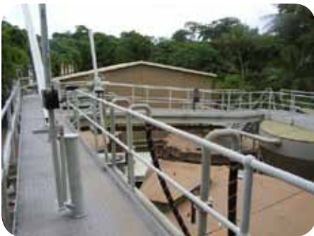
Tertiary Sewage Treatment Plant
