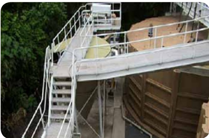
View of the Sewage Treatment Plant
