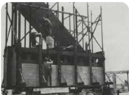
Observatory under construction
