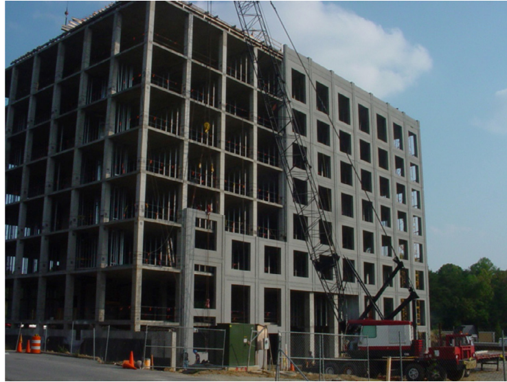
FIGURE 10. Precast concrete wall panel system in the Proximity Hotel.
