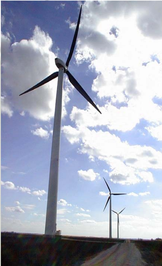
Three 750 kW Turbines at Algona, Iowa Jointly Owned by Seven Iowa Towns
