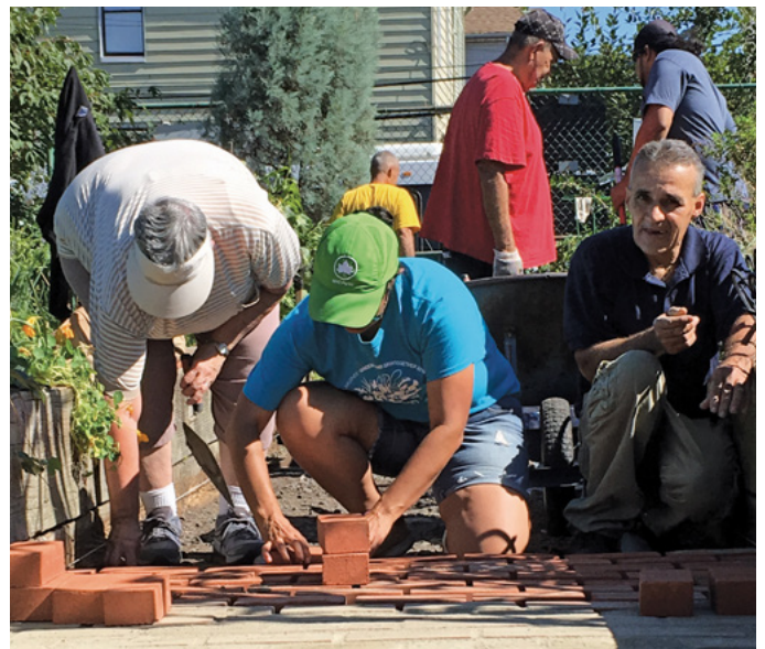
GreenThumb community gardener Angel Sepulveda demonstrating how to make a brick walkway | Photo by GreenThumb
