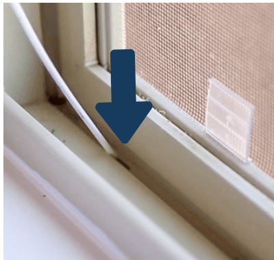
Interior weep holes.
