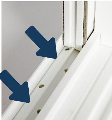
Interior weep holes.
