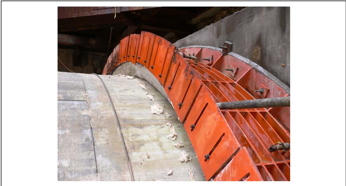
Figure 8.1 Typical Launch Seal (Courtesy of Richard Lewis)
