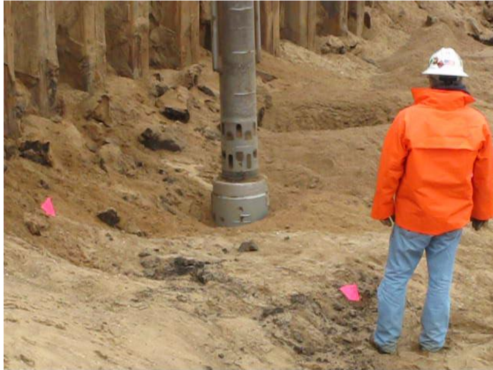
Gunderson Lutheran Hospital Parking Deck, La Cross, WI
