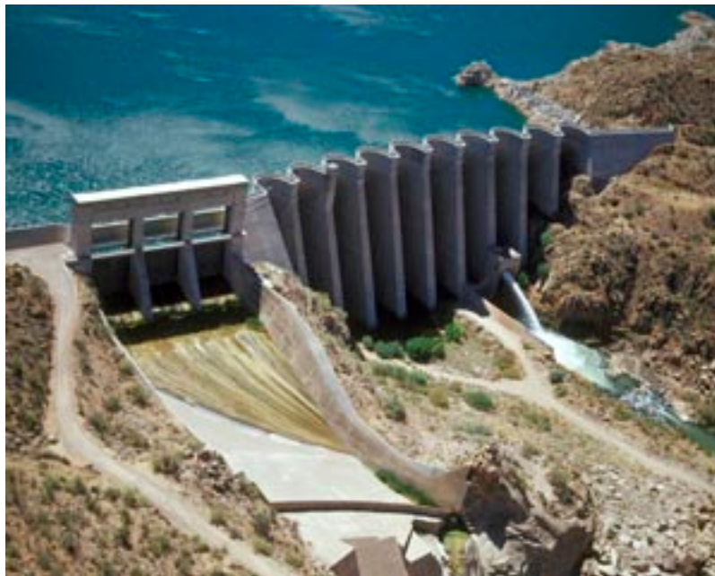
Figure 6. Concrete Multi-Arch Dam (Bartlett Dam. U.S. Bureau of Reclamation; Photo: National Park Service, 2013)
