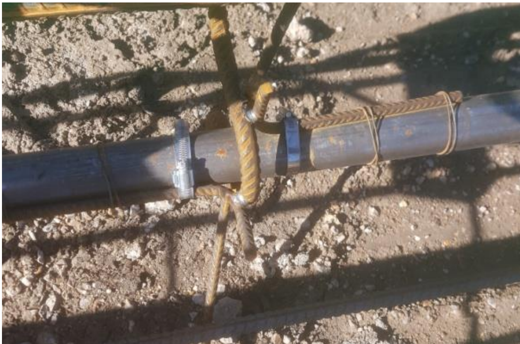
Figure 33: Securing mechanism for light weight steel tubes using jubilee clips
