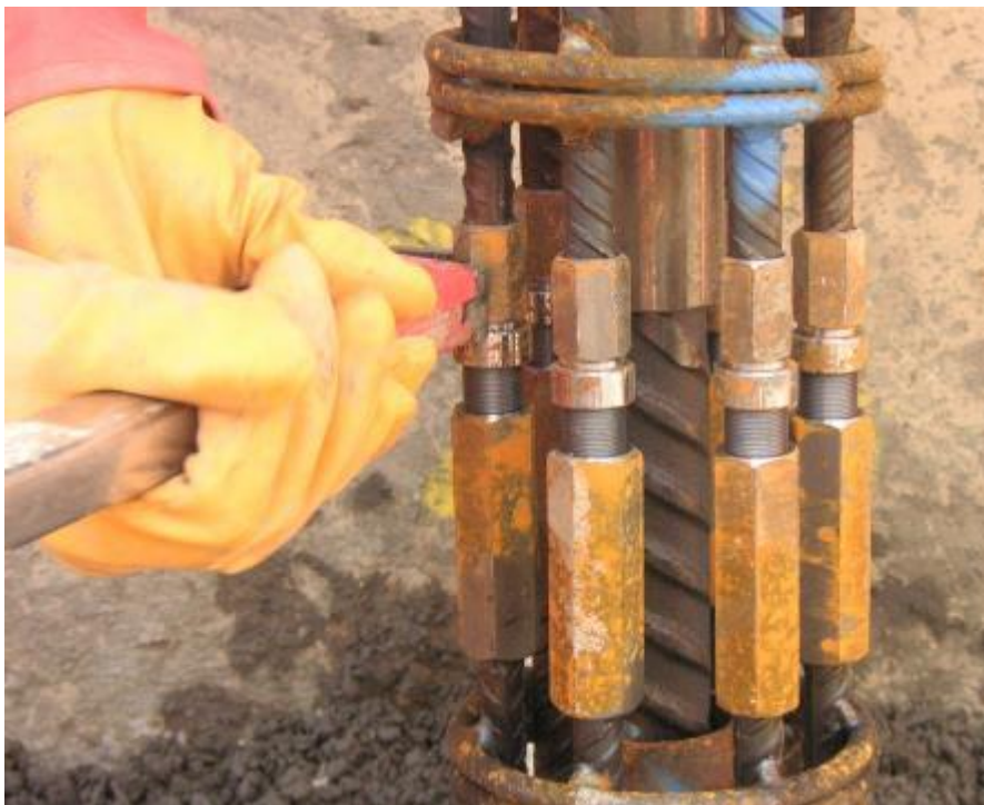
Figure 19: Torqueing up of positional couplers in mini-pile cage
