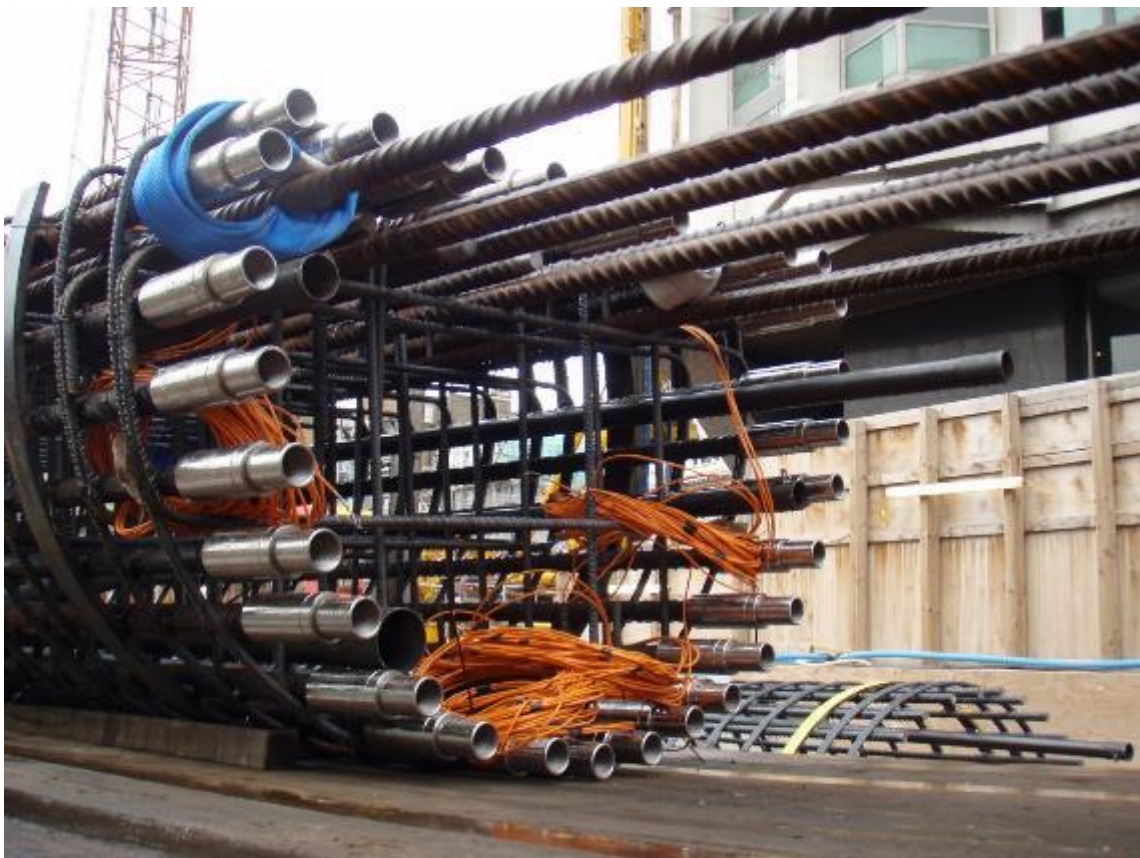
Figure 18: Use of positional couplers in pile cage
