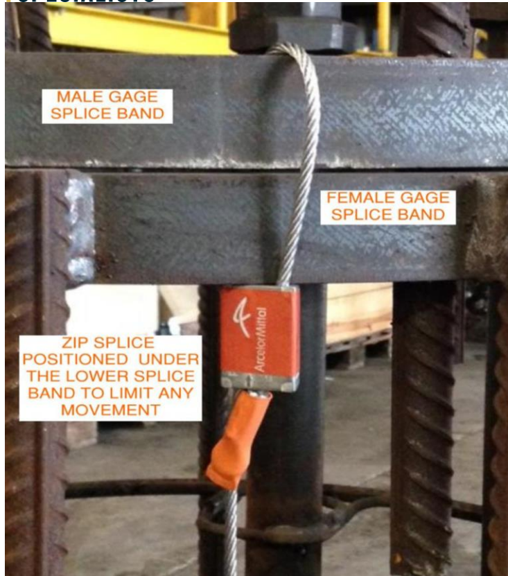
Figure 4: Zip Splice connection detail
