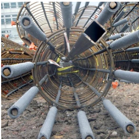
Figure 40: Square inclinometer pipe (left side – view from the top, right hand side – bottom end)
