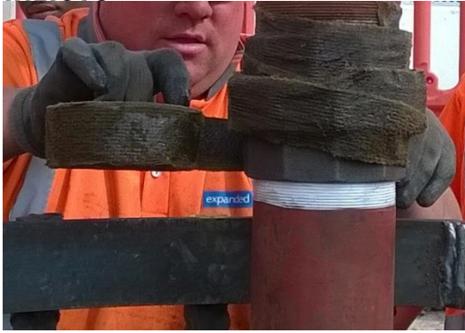
Figure 29: Use of Denso tape to enhance water tightness of joint
