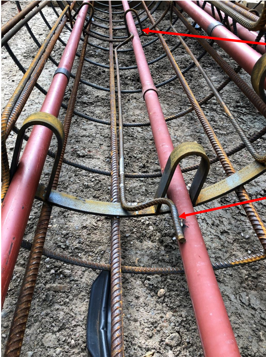
Figure 27: Close up of slider/stopper and locator bracket
