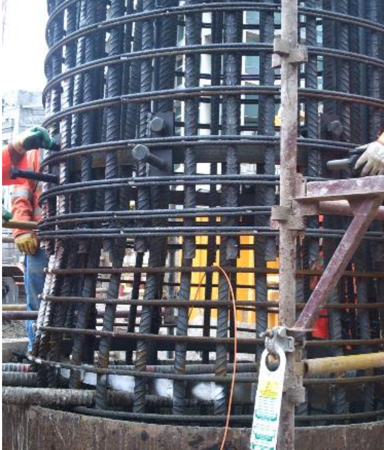
Figure 12: Safe Splice connection on pile cage
