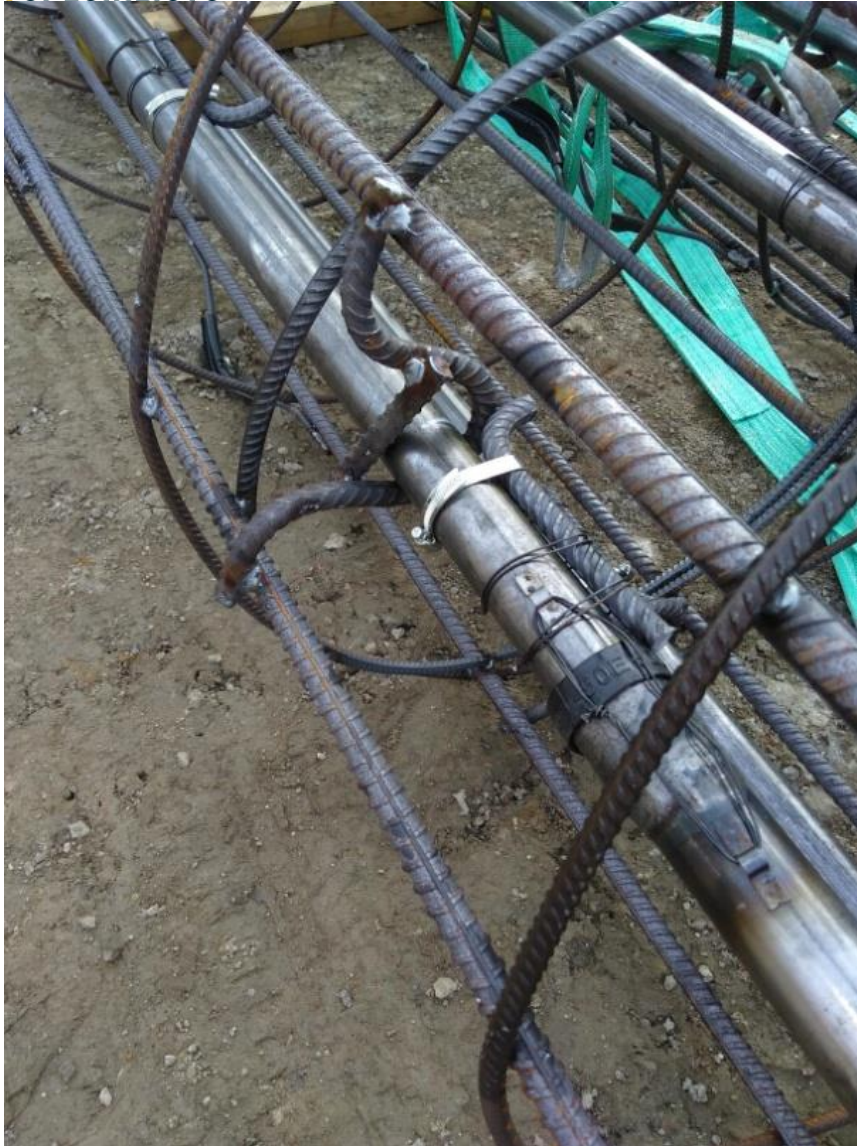
Figure 34: Securing mechanism for light weight steel tubes using tie wire
