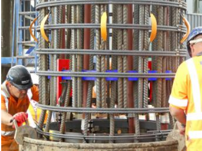
Figure 14: Engaged Superlatch system (red) and splicing band (blue) on rotary cage
