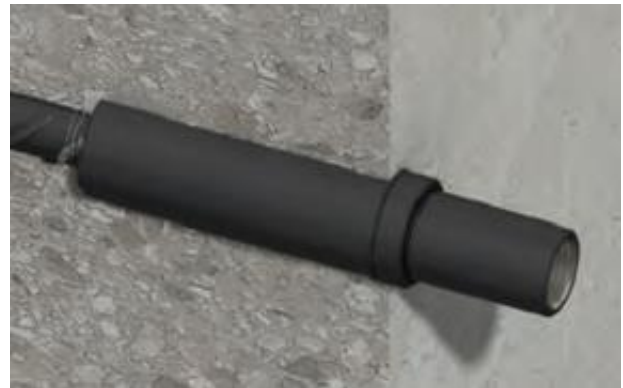
Figure 17: Ancon tapered thread positional coupler
