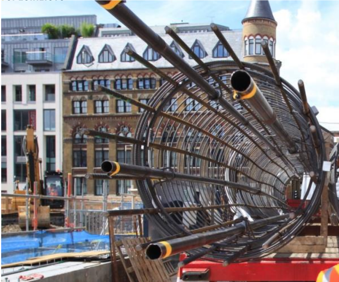
Figure 23: Top tube has slid out during transport of the cage
