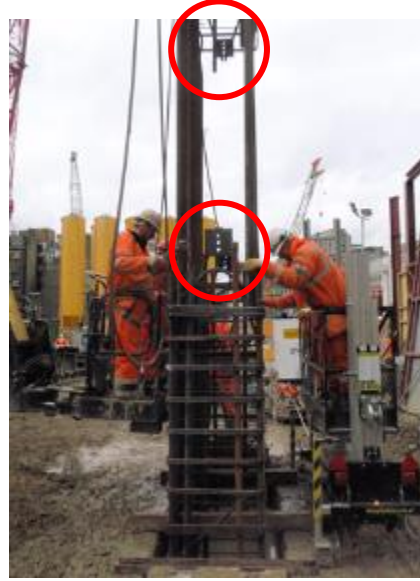
Figure 21: Splicing of diaphragm wall cages using the fish plate system
