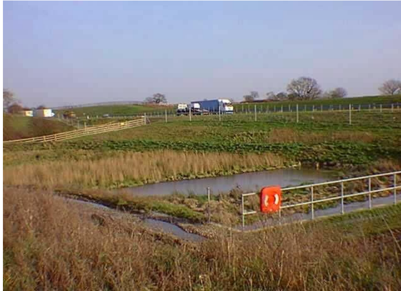
Plate 2. Overview of Pond B looking towards the inlet, alongside the A34 (Newbury Bypass). Surface flow constructed wetland and balancing pond
