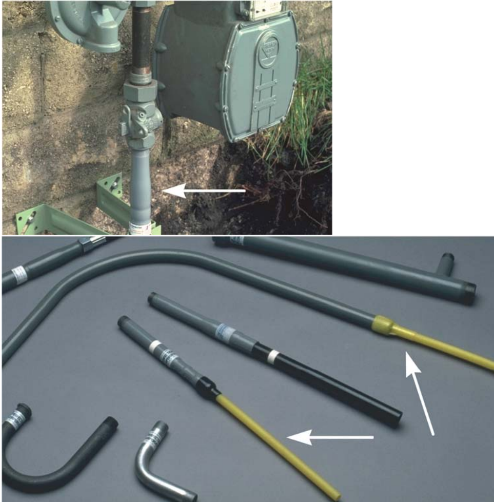
Figure VI-17: Anodeless risers
