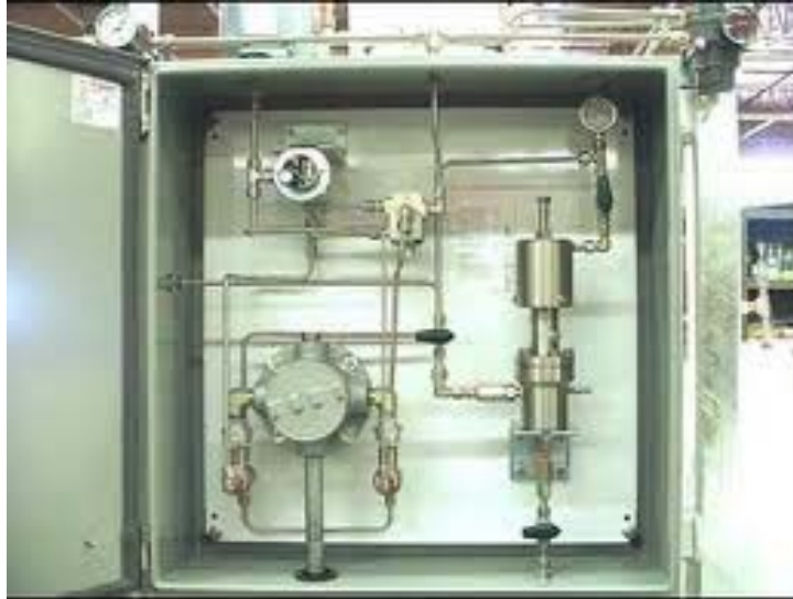
Figure IV-13: Injection-Type Odorizer
