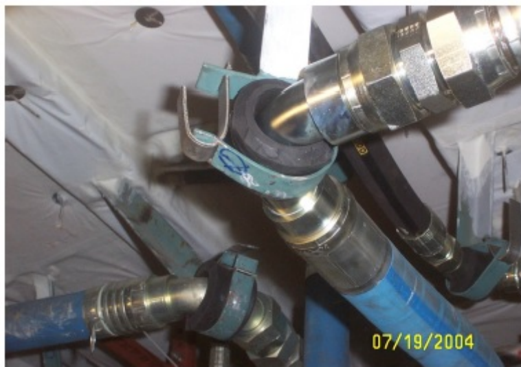
FIGURE 7 Typical Resilient Pipe Support
