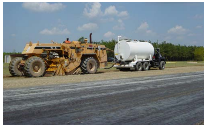
Figure 1.17. FDR construction of airport runway
