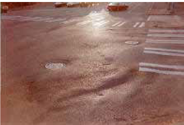
Figure 3.16. High-severity shoving
