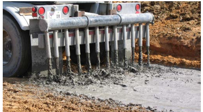
Figure 6.6. Cement slurry application
