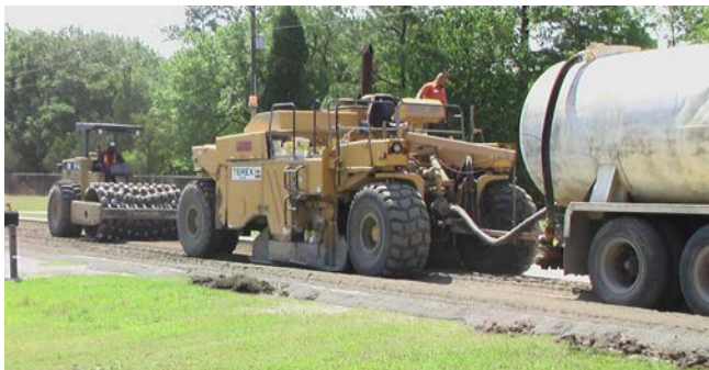
Figure 6.8. Water truck supplying road reclaimer during mixing operations
