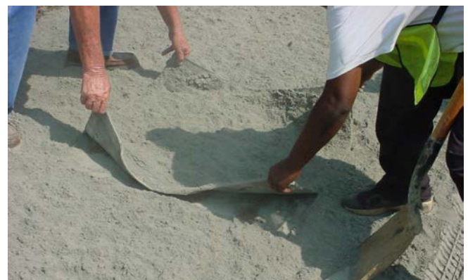
Figure 7.2. Cement application rate verification
