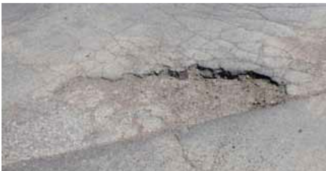
Figure 3.12. High-severity pothole
