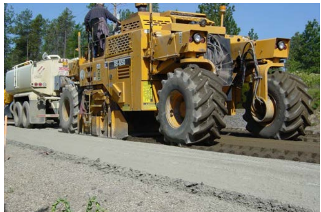
Figure 1.11. Full-depth reclamation train with water truck (left) and reclaimer
