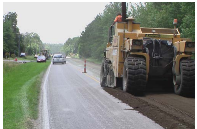
Figure 6.13. Pulverization of existing asphalt roadway
