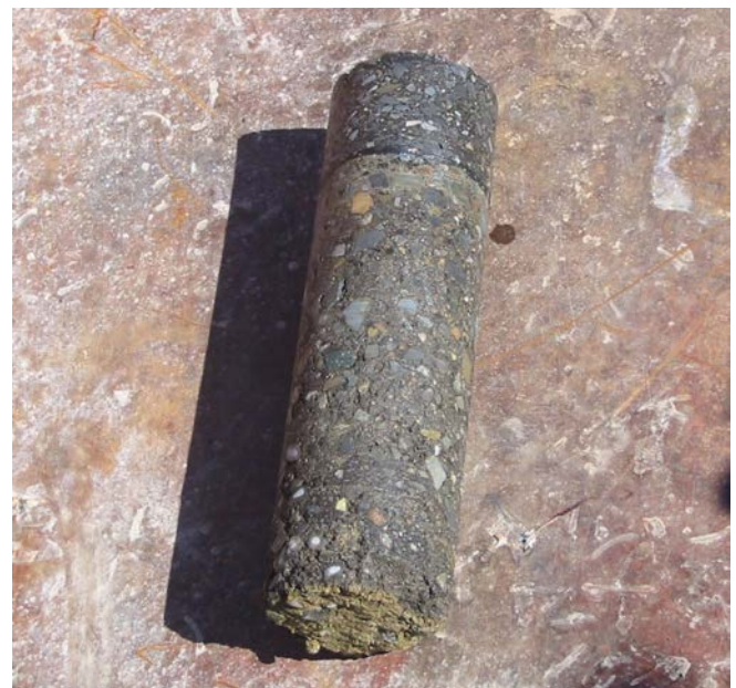
Figure 7.8. Core from a completed FDR project
