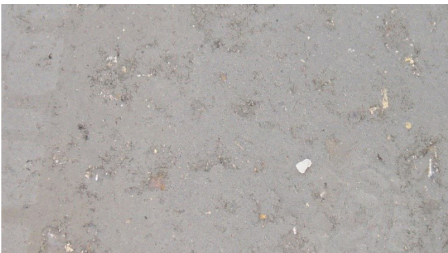
Figure 4.15. Properly prepared FDR surface for a bonded concrete overlay
