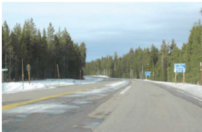
Figure 1.15. US 20 in Idaho after FDR construction
