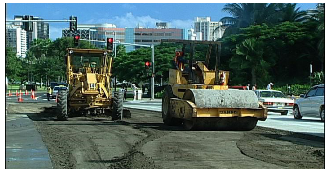
Figure 6.18. Compaction and final grading operations
