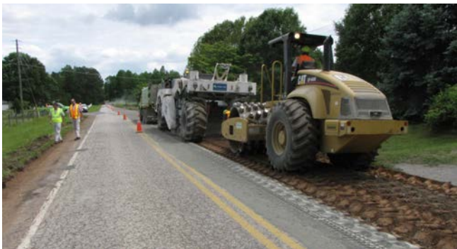
Figure 6.9. Tamping-foot roller behind reclaimer
