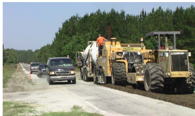
Figure 6.20. Full-depth reclamation while maintaining traffic
