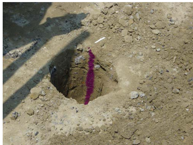
Figure 7.5. Checking depth of cement stabilization with phenolphthalein
