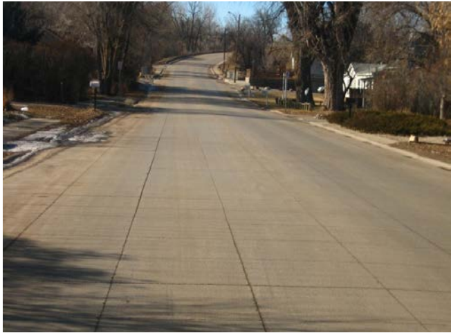
Figure 4.14. Bonded concrete overlay of FDR layer
