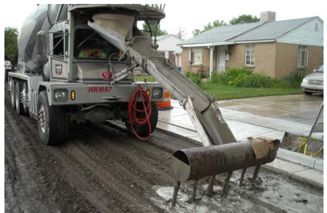
Figure 6.7. Cement slurry application on grade using a concrete ready mixed truck
