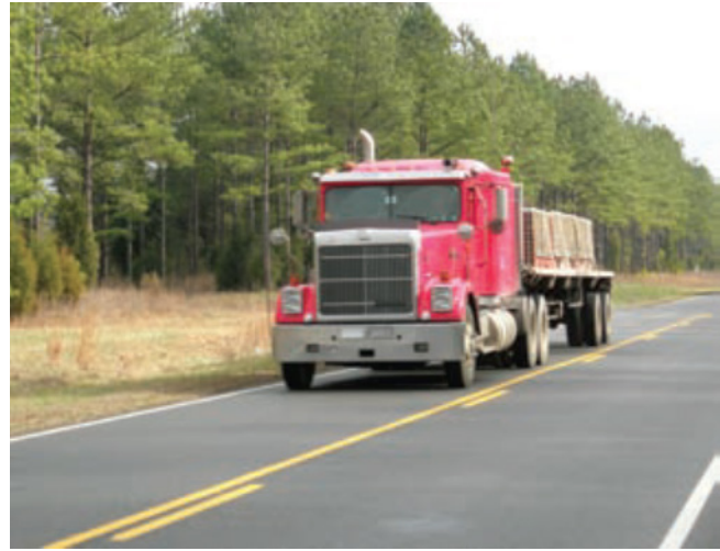
Figure 4.1. Well designed and constructed FDR project in South Carolina
