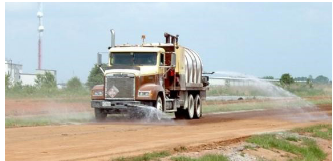
Figure 6.19. Water truck spraying on compacted FDR layer
