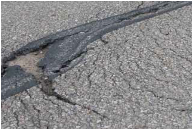
Figure 3.15. Low- to medium-severity shoving
