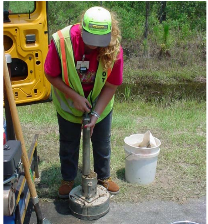
Figure 7.7. Proctor test during construction
