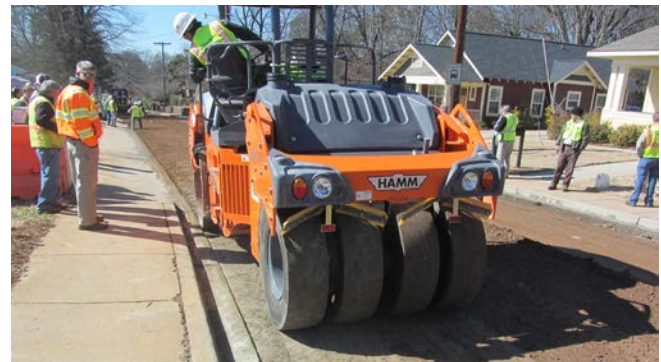
Figure 6.10. Finish rolling using pneumatic tire roller
