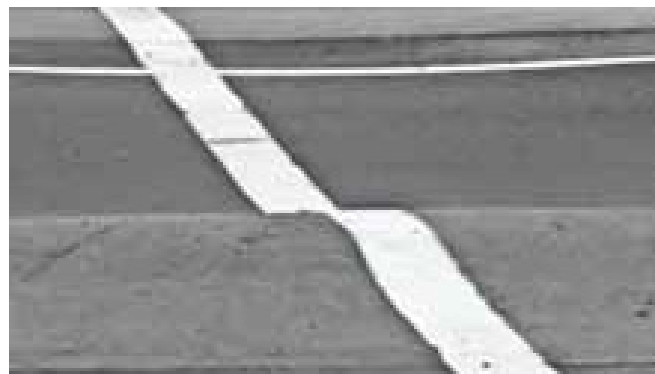
Figure 3.14. High-severity rutting
