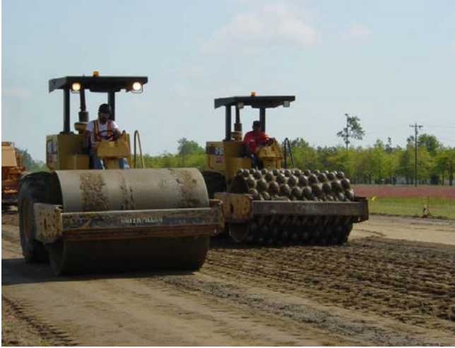
Figure 1.12. Final compaction of FDR base with a tamping roller (right) and a smooth-wheeled vibrating roller
