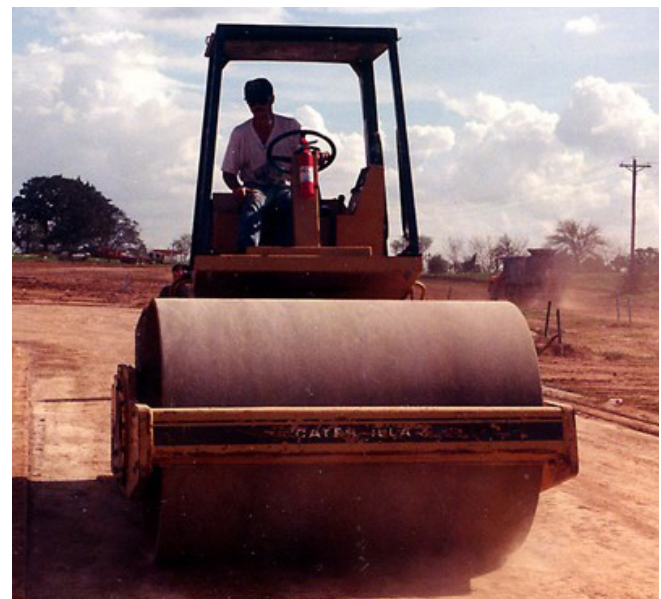
Figure 6.11. Smooth-drum vibratory roller
