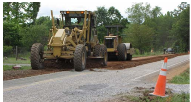
Figure 6.15. Grading of pulverized FDR mix
