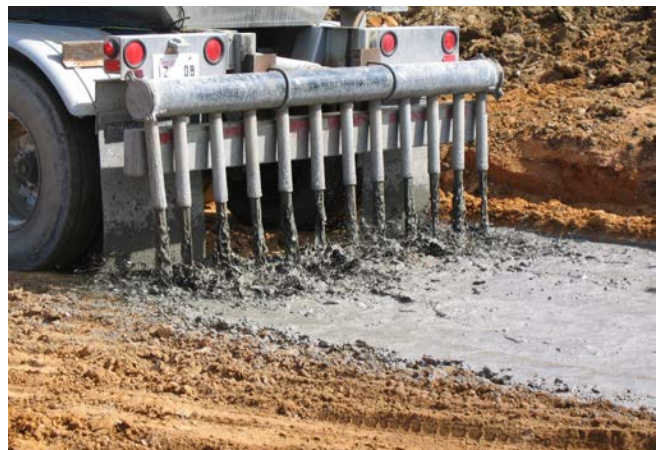
Figure 1.10. Application of cement slurry to pulverized mix
