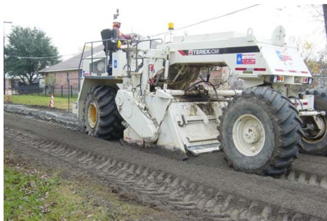
Figure 6.17. Cement slurry mixing operations
