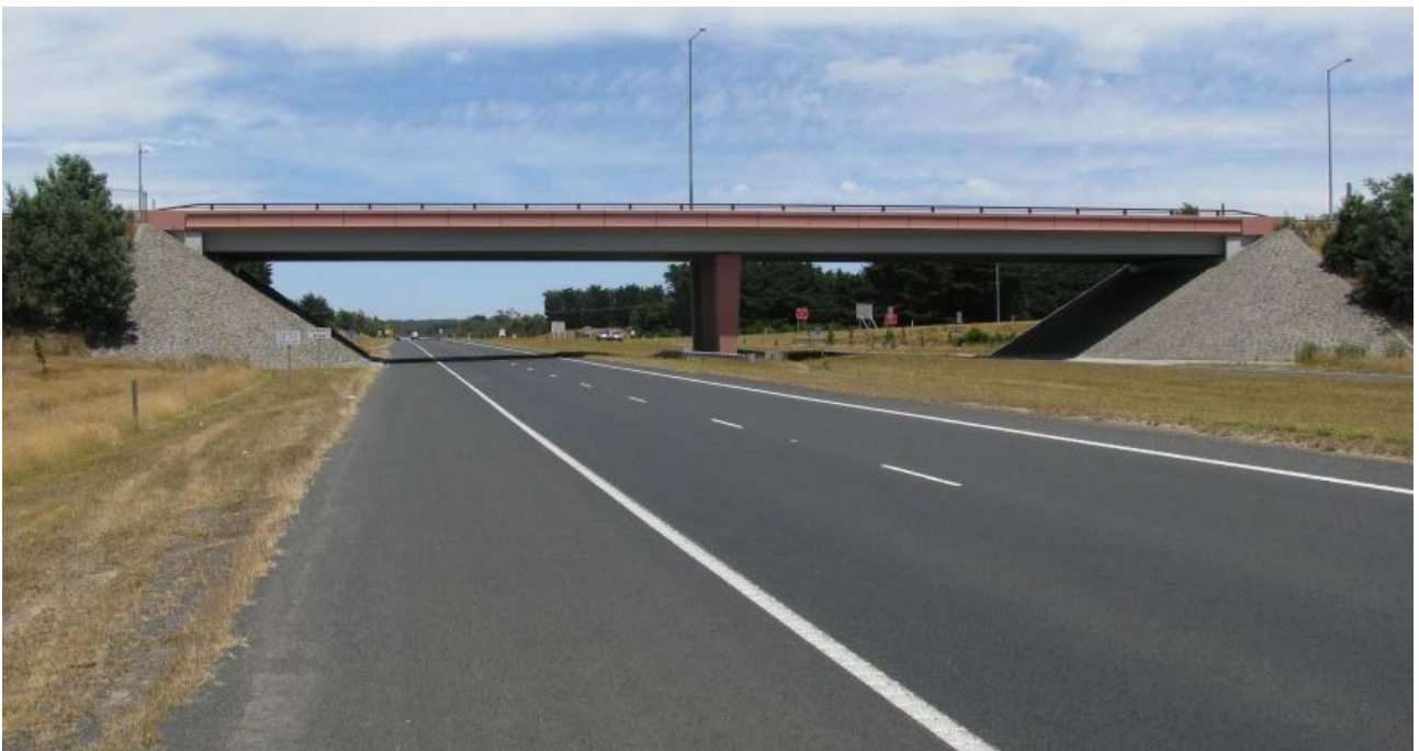
Figure 4.2: Open-end or spill-through bridge abutment
