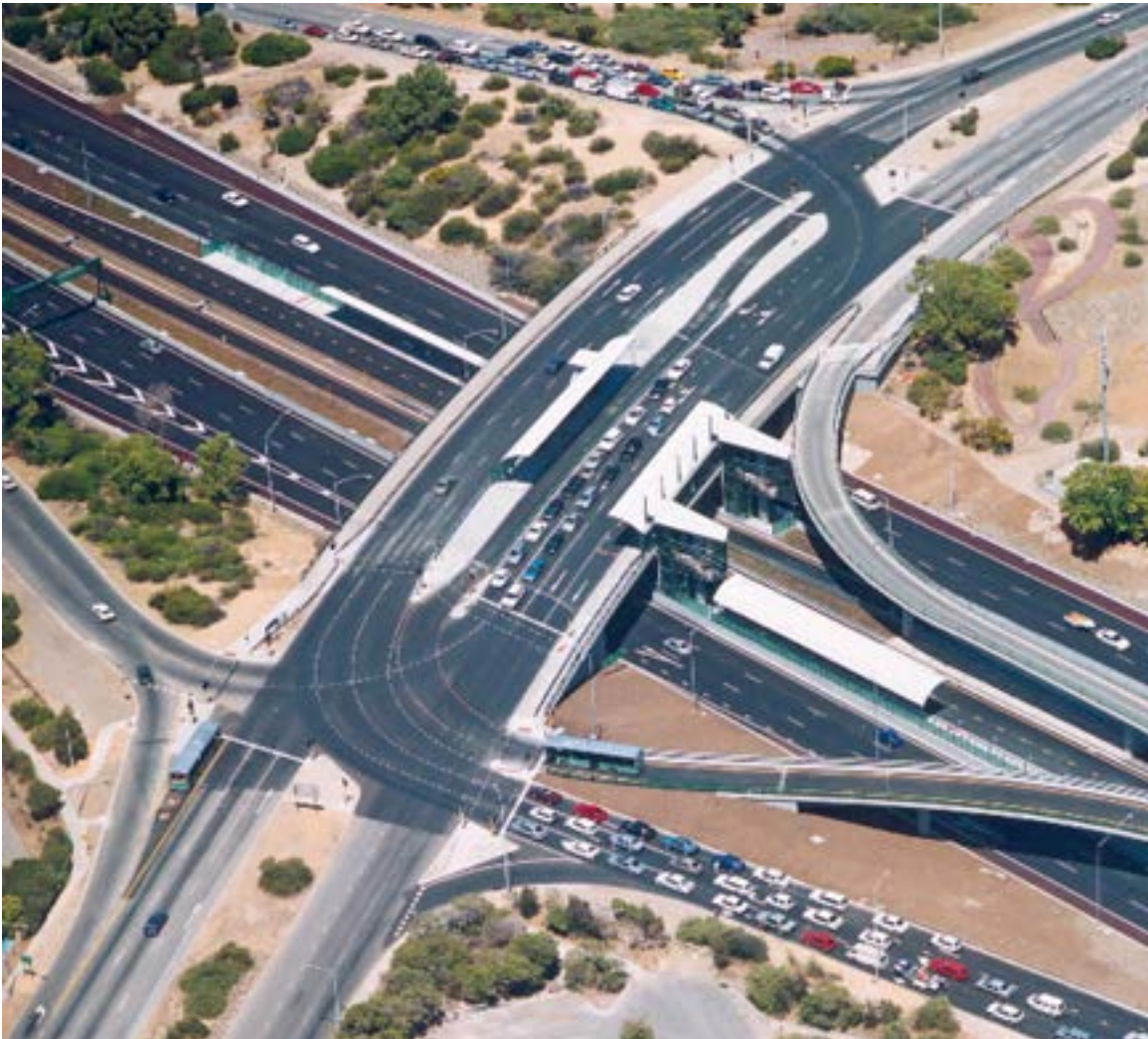
Figure 2.1: Dedicated freeway entry/exit ramps for the Kwinana Freeway busway (Canning Highway Interchange)
