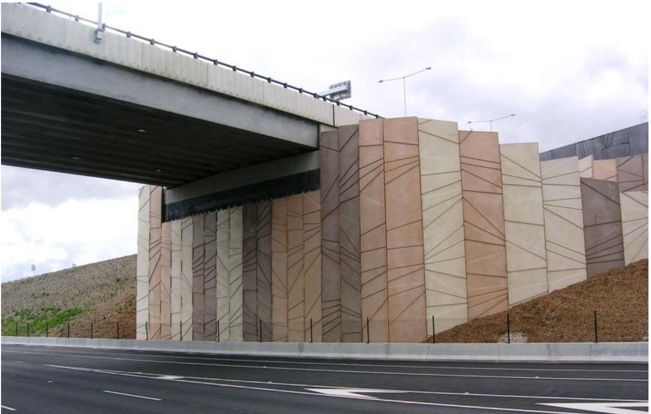
Figure 4.1: Solid-end (or vertical) bridge abutment
