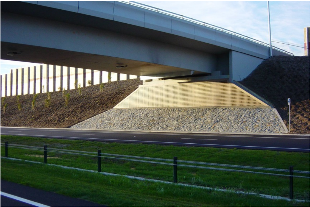
Figure 4.3: Combination of solid-end and spill-through bridge abutment
