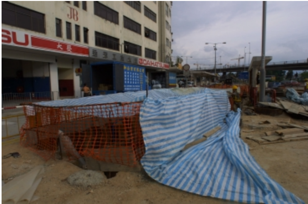
Plate B7 – Tarpaulin cover secured against wind for wider trenches
