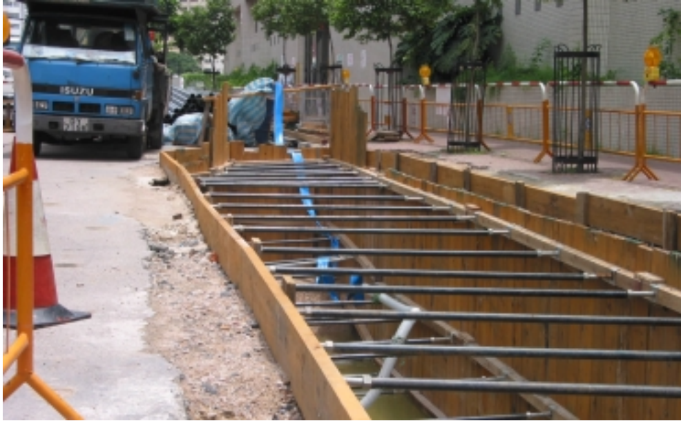
Plate A3 – Timber support for deeper excavation
