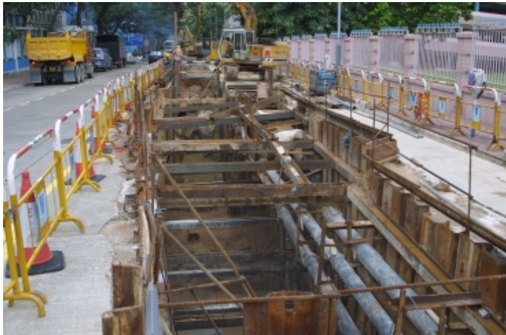
Plate A5 – Steel sheet pile support
