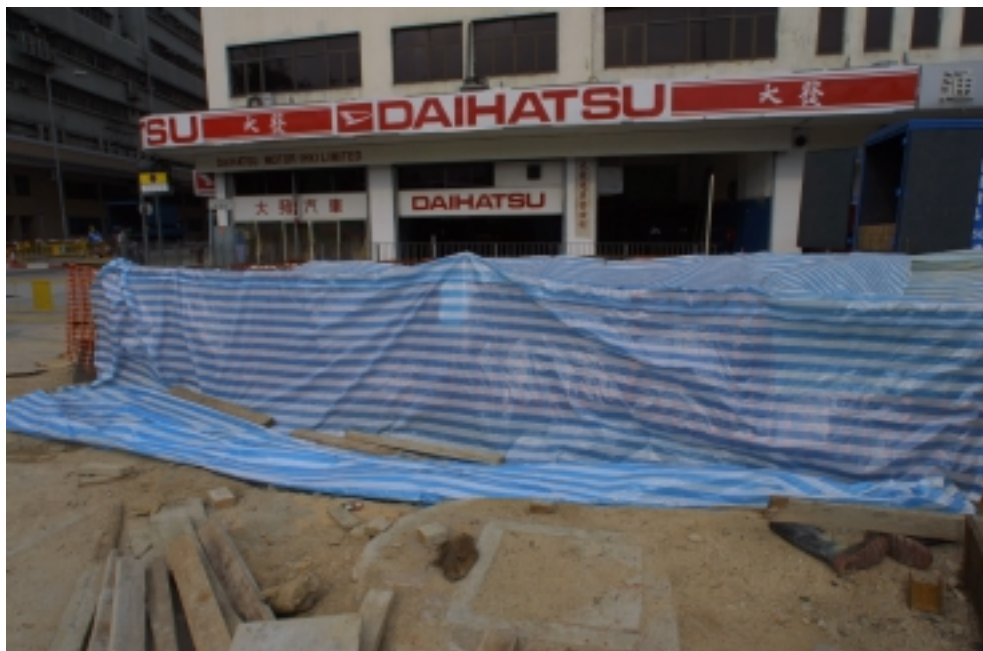
Plate B8 – Tarpaulin cover secured against wind for wider trenches
