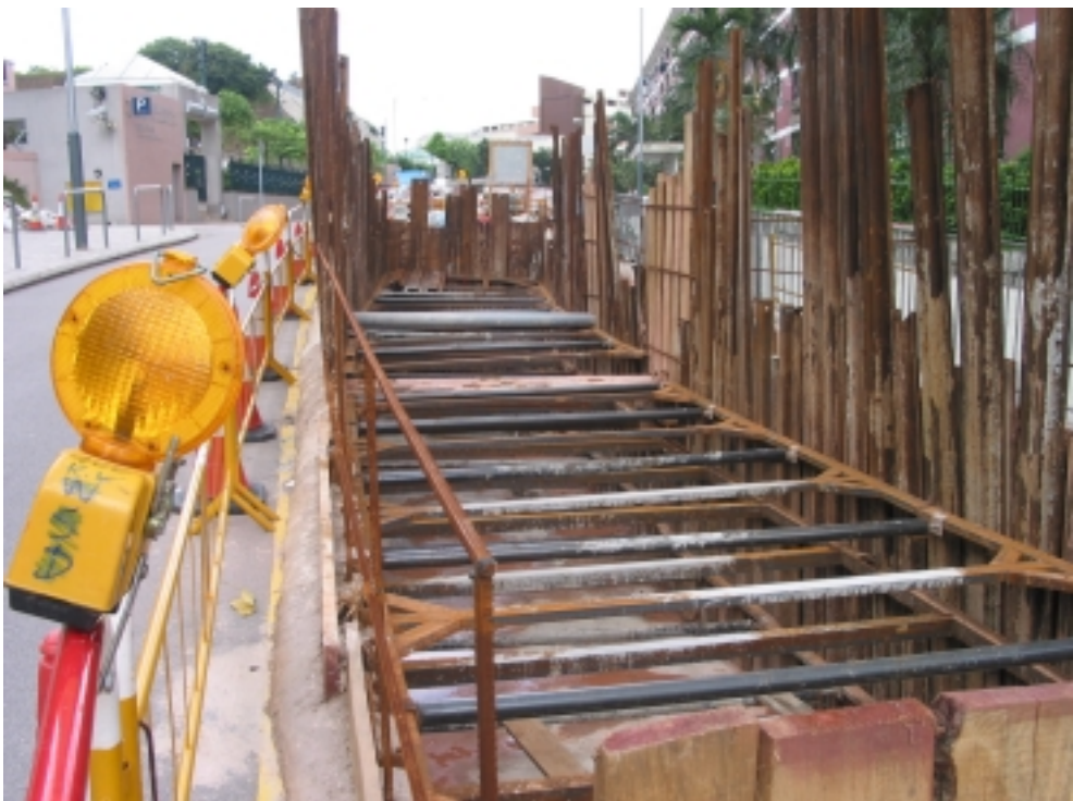
Plate A4 – Steel sheet pile support
