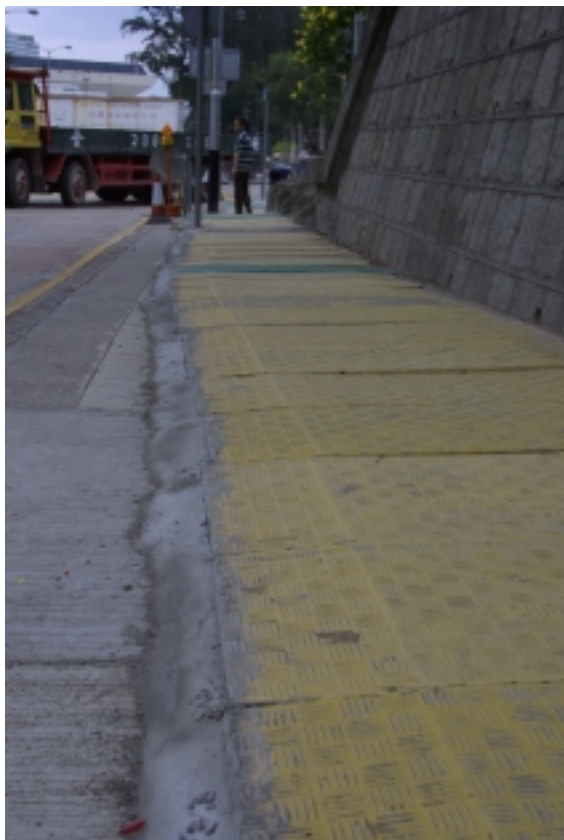
Plate B2 – Typical pedestrian crossing trench opening which is also effective for preventing surface runoff and infiltration of rainwater
