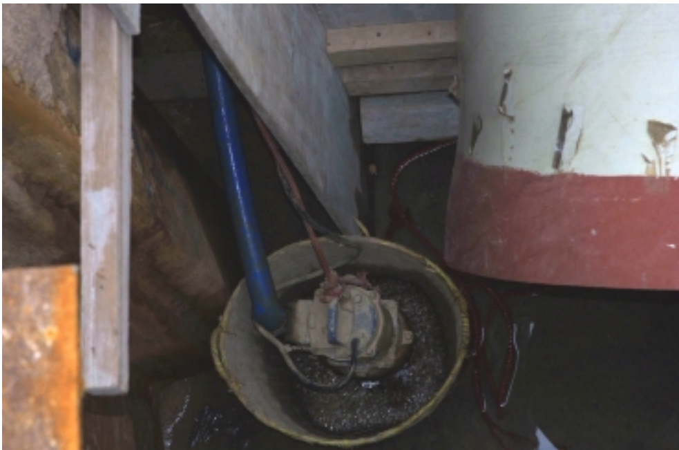
Plate B6 – Pumping provided
