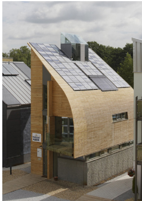
Image 9: Vacuum tube solar collector and PV panels (Kingspan lighthouse)
