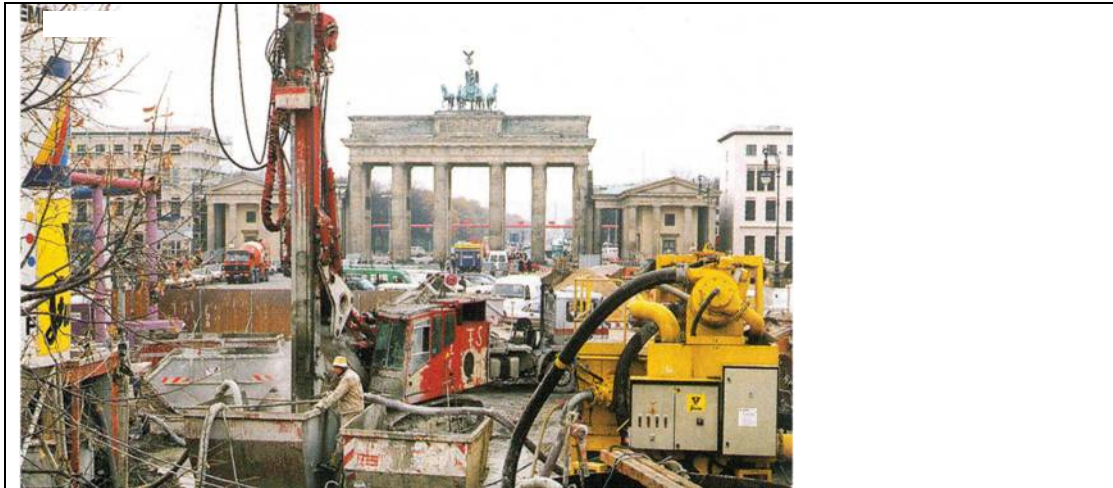
Fig. 1: Construction work close to the Brandenburg Gate in Berlin, Germany
