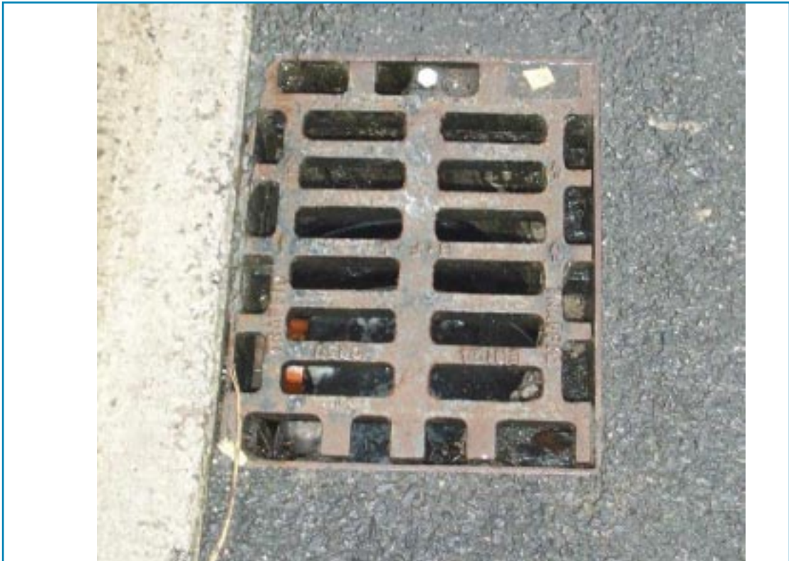
Photo 3.3 Side entry gully – facilitates cyclists
