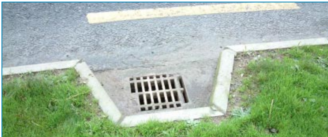
Photo 4.1 Kerbs & Gully (inset into verge)
