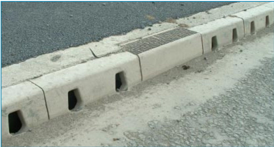
Photo 4.3 Combined Kerb and Drainage Block
