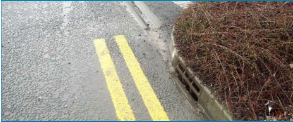
Photo 3.3 Side entry gully – facilitates cyclists
