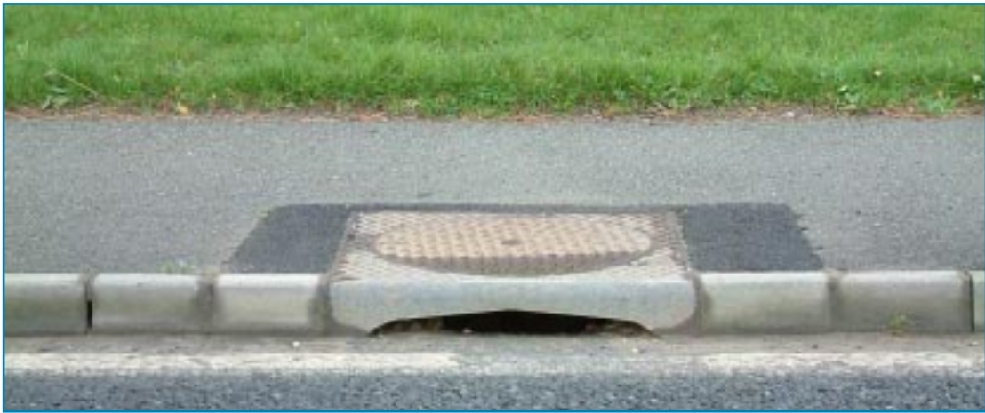
Photo 4.2 Side Entry Gully
