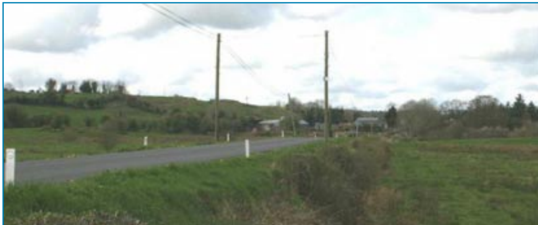
Photo 4.7 Over the Edge Drainage
