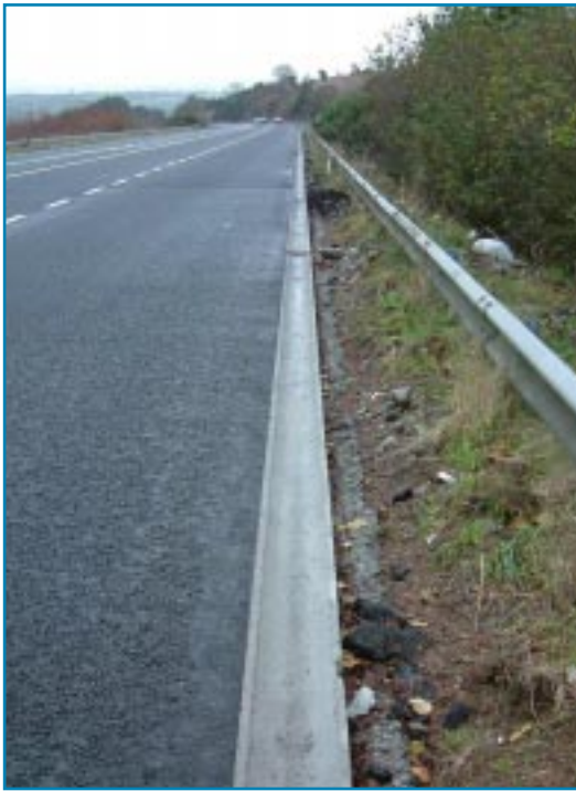
Photo 4.5 Surface Water Channel
