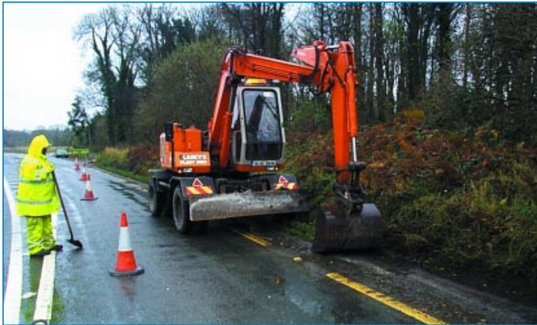
Photo 3.7 360 degree rubber wheeled hydraulic excavator
