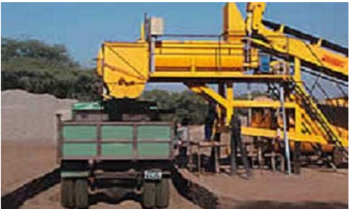
BLANKET MATERIAL BEING LOADED INTO TRUCK
