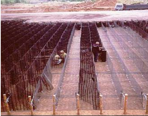
Geocell – Fabrication
