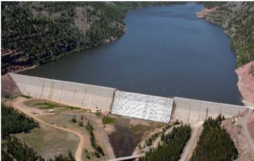
Figure 2: Upper Stillwater Dam located on Rock Creek in Utah.
