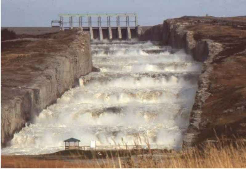
Figure 4: Spillway of the Robert Bourassa dam in Quebec, Canada. Excavated from rock, this unlined channel is almost 3280 ft (1 km) in total length, there are 10 steps each 32.8-ft-high (10-m) with tread lengths of up to 590 ft (180 m), and width of 400 ft (122 m), design discharge is 574,000 ft 3 /s (16250 m 3 /s).
