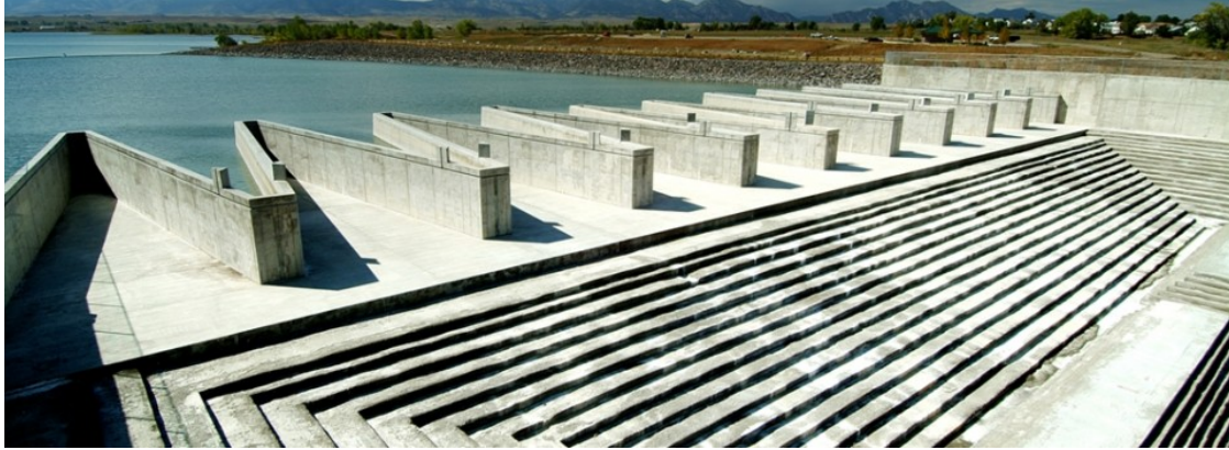
Figure 7: Labyrinth weir leading into a stepped chute, Standley Lake, Westminister, Colorado.
