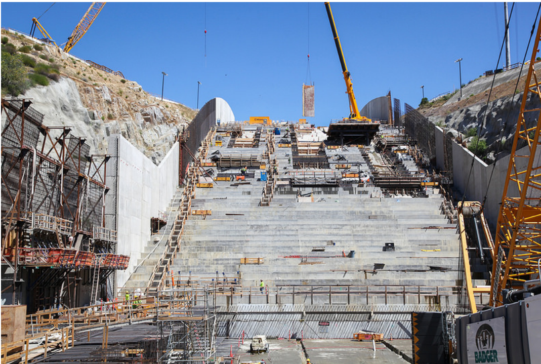
Figure 11: Auxiliary spillway on the Folsom Dam, California under construction, April 2015.
