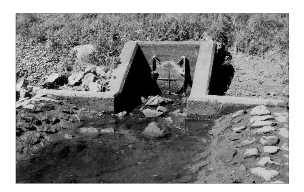
through the dike with a flap gate at the waterside outlet and may have trash racks fitted at the inlet and/or the outlet.
