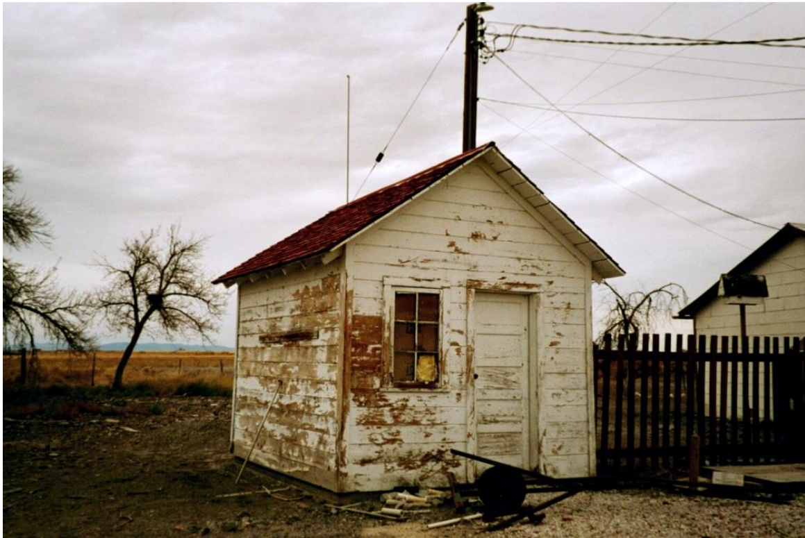
Figure 6. ASSOCIATED RESOURCE: Pumphouse, ranch property, Stillwater NWR (USFWS).
