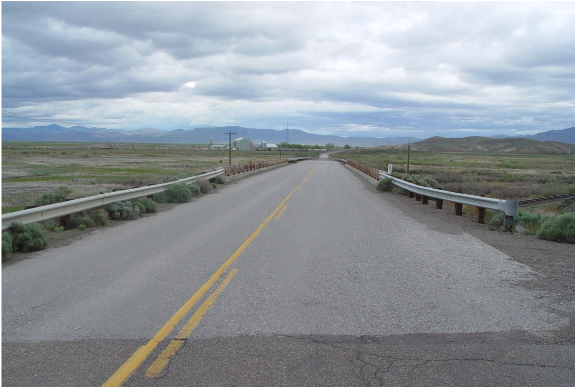
Figure 18. Segment of the Old Victory Highway, also known as US 40, near Dunphy, Elko County. This road has been continually maintained but is on its original alignment and has three 1940s era bridges on it (Cliff Creger, 2012)
