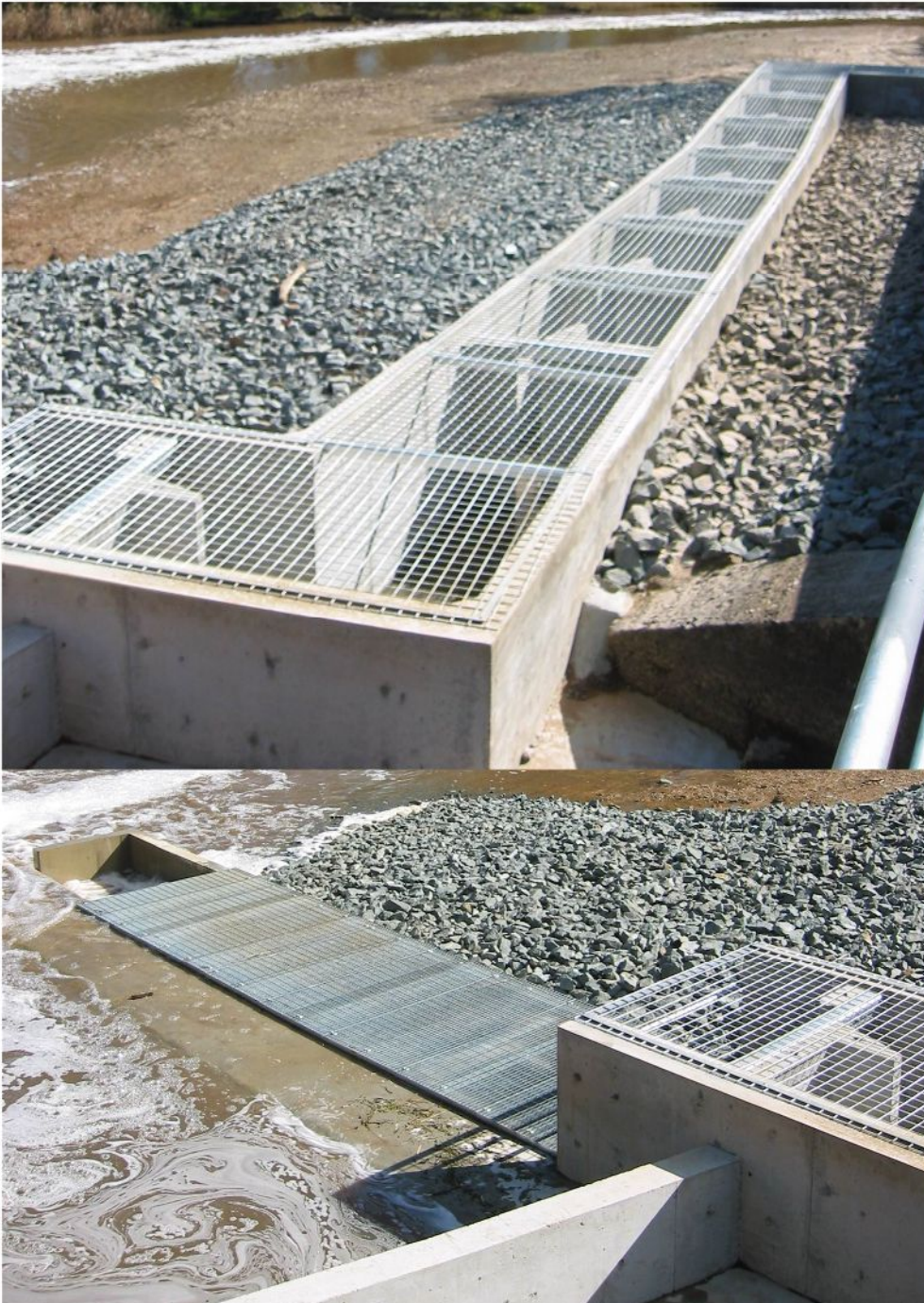
Figure A1.2: Vertical-slot fishway, Broken River.
