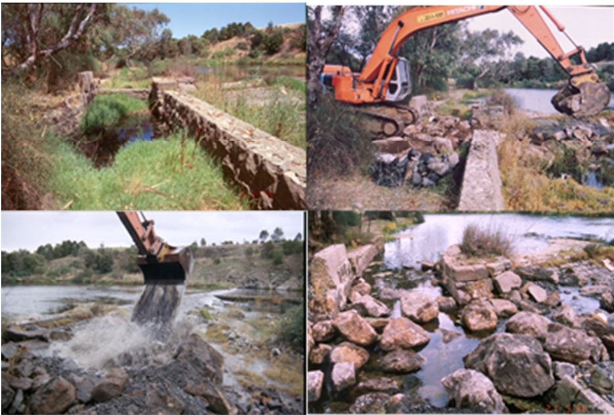
Figure A1.1: Barrier removal, Barwon River.
