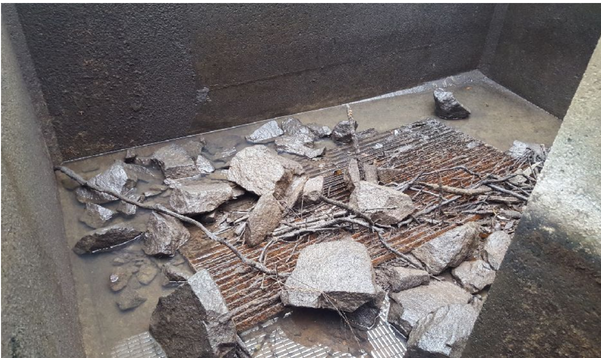
Figure 4.3: Example of a vertical-slot fishway without a maintenance schedule. The outcome can alter cell volume and hydraulics, thus reducing functionality of the fishway and so fish passage.
