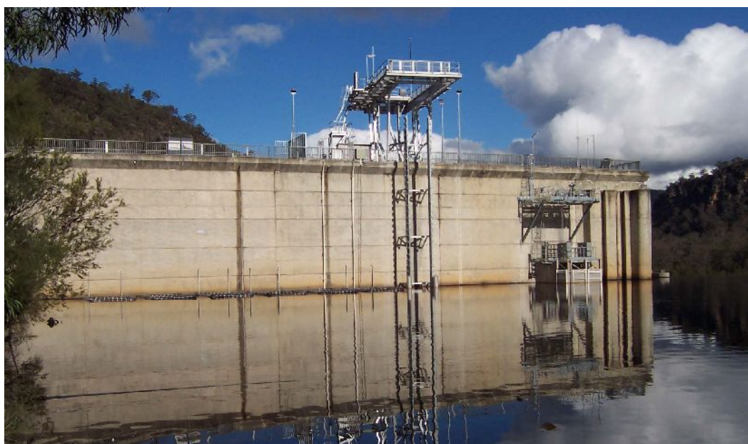
Figure A1.5: Ascending hopper lift on Tallowa Dam, Shoalhaven River.
