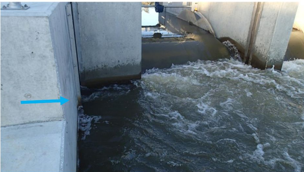
Figure 4.1: Fishway entrance flow (blue arrow), showing high integrity of flow and low recirculation within 0.5 m of the entrance (photo: M. Mallen-Cooper)
