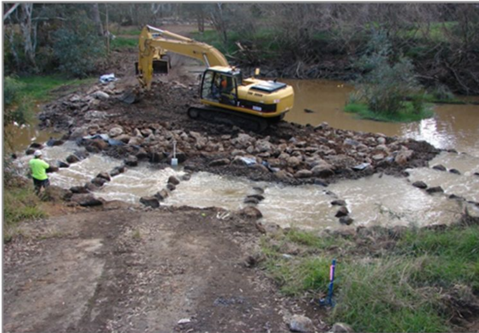
Figure A1.4: Two lateral-ridge-rock fishways: a full-river-width design at Pollocksford Weir on the coastal Barwon River (top) and a partial-width design on Sugarloaf Creek near Puckapunyal (bottom). (photos: I. Stuart)
