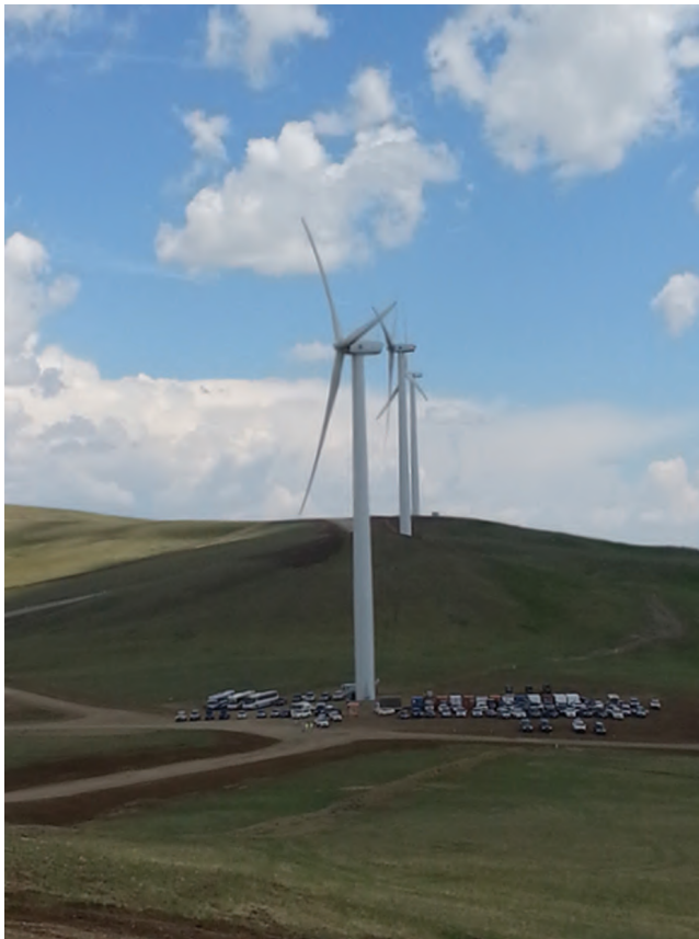
Salkhit wind farm in Mongolia.
