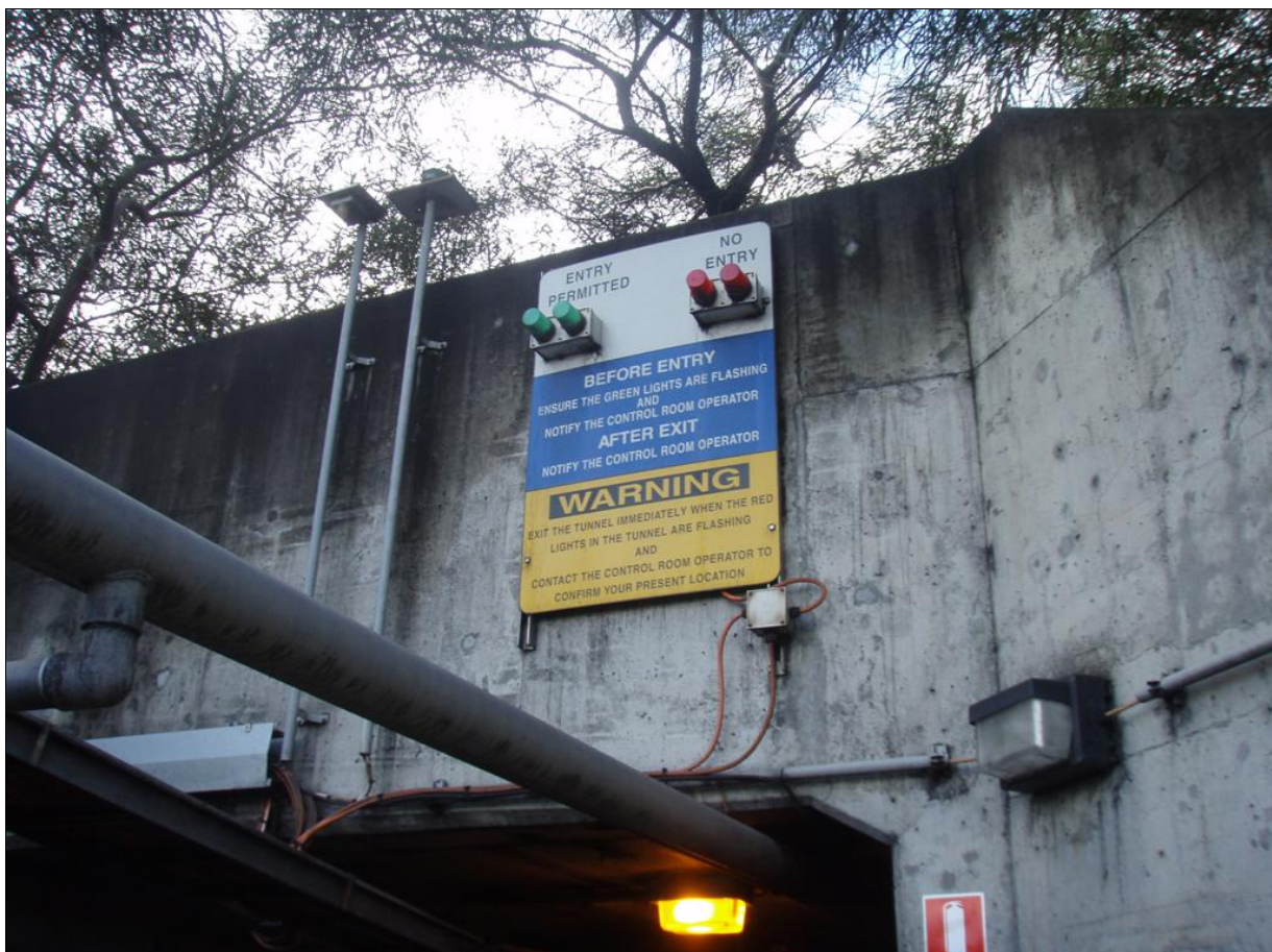
Figure 9. Entrance to reclaim tunnel.
