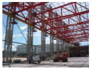
Designing a structure so that work does not need to be performed at height will prevent fall incidents e.g. lifting and erection of a hangar's roof truss.
