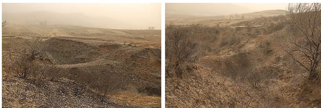
Figure 7. Typical soil check dams (photos taken by Dr. X.Y. Zhang in May 2018, Zhangwu County, Liaoning Province).
