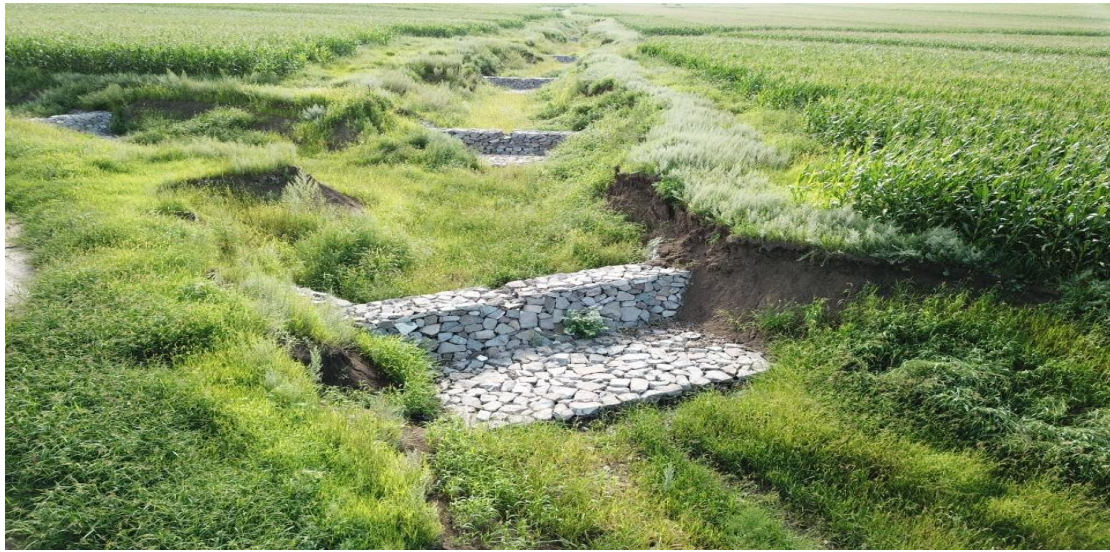
Figure 3. Engineering system for gully control (photo taken by Dr. X.Y. Zhang in July 2018, Arongqi County, Inner Mongolia Autonomous Region).
