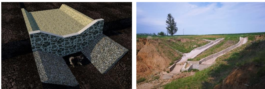
Figure 5. Masonry drop structure for medium-sized (left) and large-sized gullies (right) (photos taken by Dr. X.Y. Zhang in June 2018, Hailin County, Heilongjiang Province).
