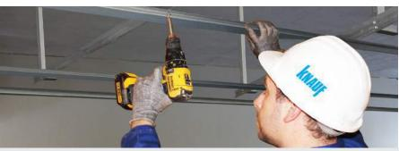
6 Screw spacing for fixing of the boards : max. 300 mm.
