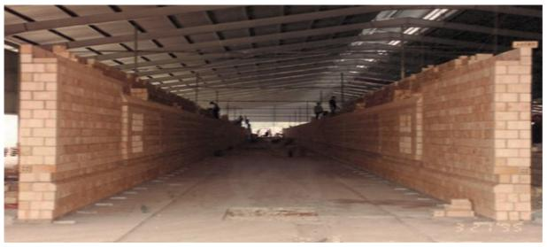
Mullite insulation brick: temperature 1400°C,  $AL_2O_3 \ge 56\%$ ,  $Fe_2O_3 \le 0.7\%$ , bulk density  $0.9g/cm^3$ , Cold crushing strength  $\ge 40kgf/$  cm<sup>2</sup> ,thermal conductivity W/(m.k) , average temperature  $(350\pm25^{\circ}C) \le 0.33$ , Re sintering shrinkage  $\le 0.6\%$
