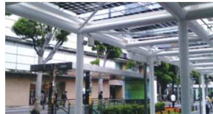
Structure made of steel pipes processed by the 3D FABRI GEAR 300
