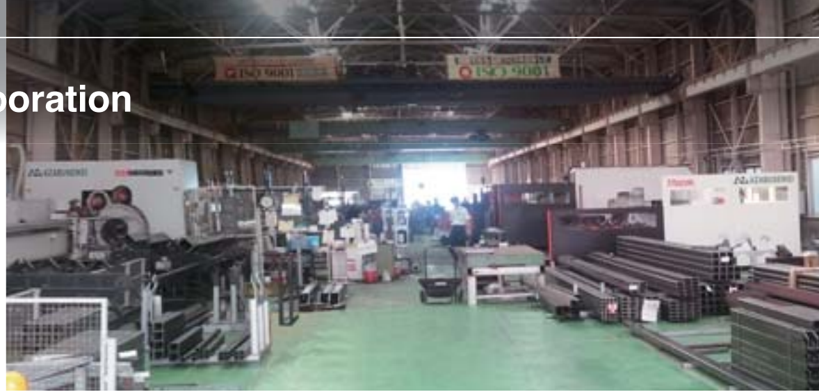
Second 3D FABRIGEAR was installed in July this year
