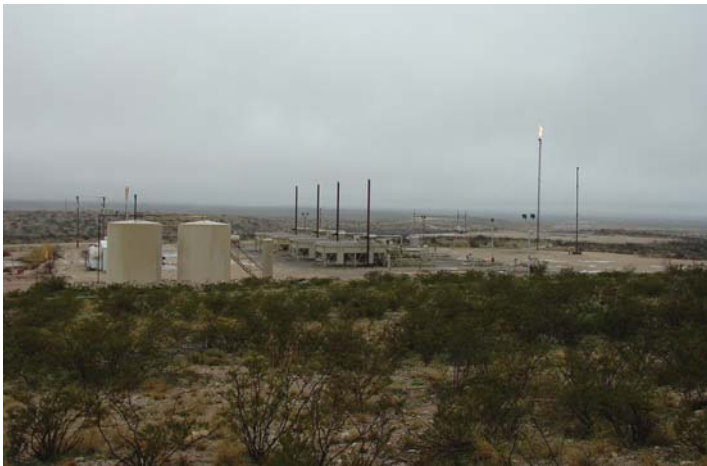
Figure 46. Example of the large footprint left by the variety of support facilities at a gas production area near Carlsbad, New Mexico (Photo courtesy of NMDGF).
