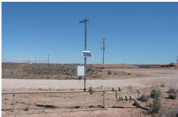
Figure 43. Remote monitoring stations can be used to minimize traffic at the well site. (Photo courtesy of NMDGF)
