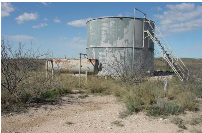
Figure 48. Failed reclamation of an oil well site. Support structures should be removed during reclamation. (Photo courtesy of NMDGF)
