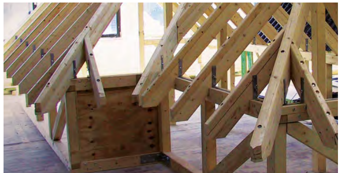
Timber pitched-roof construction
