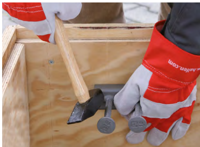
Nail the HALFEN Cast-in channel to the formwork
