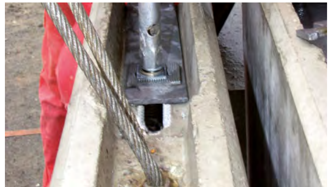
HVL-System in precast building components
