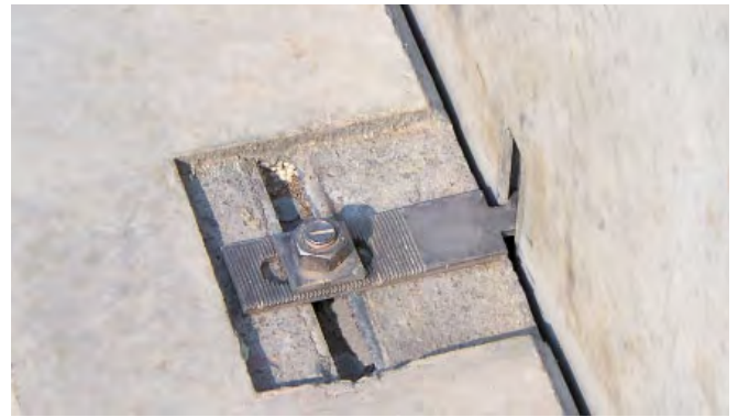
HALFEN HKZ Restraint tie with serrated washer
