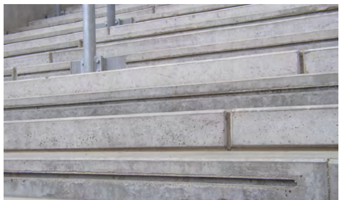
Fixing of safety rails, Rheinenergiestadion Cologne
