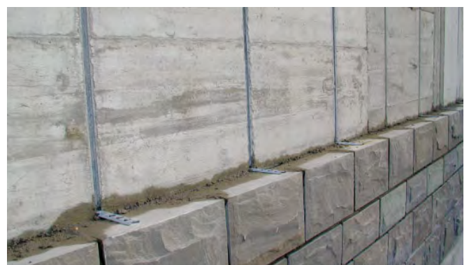
HALFEN ML Brick-tie anchor system
