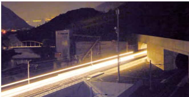
Lötschberg-Base tunnel, Switzerland
