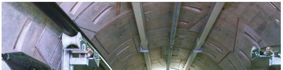
Curved HALFEN Cast-in channels in tunnel segments
