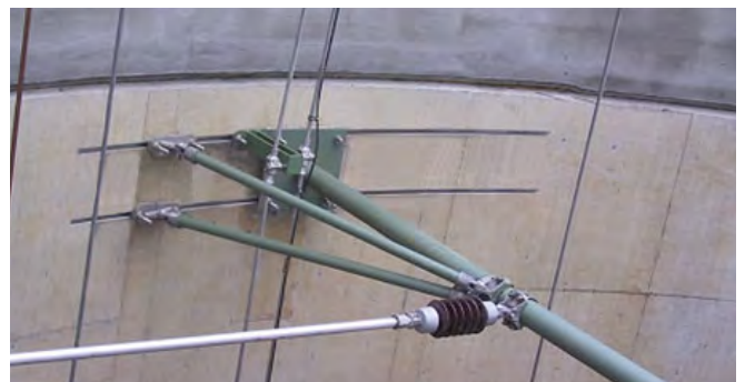
Fixing of overhead cables in railway tunnels
