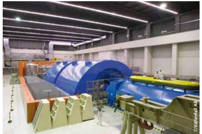
Turbine block in a nuclear power plant
