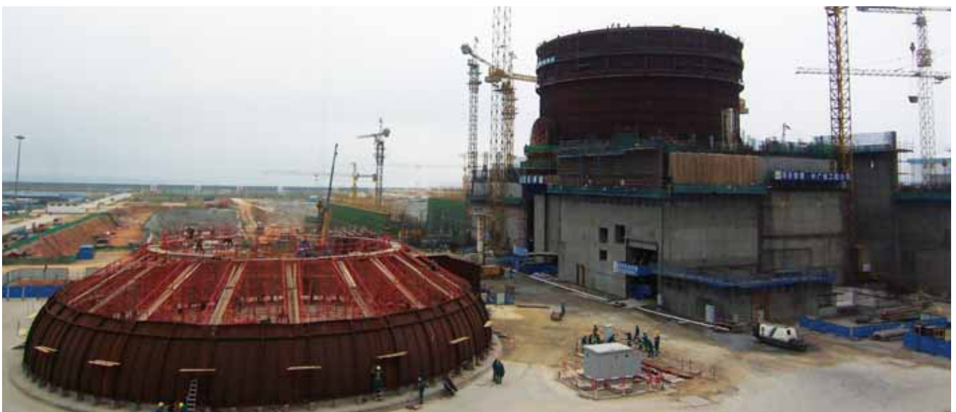
Nuclear power plant under construction
