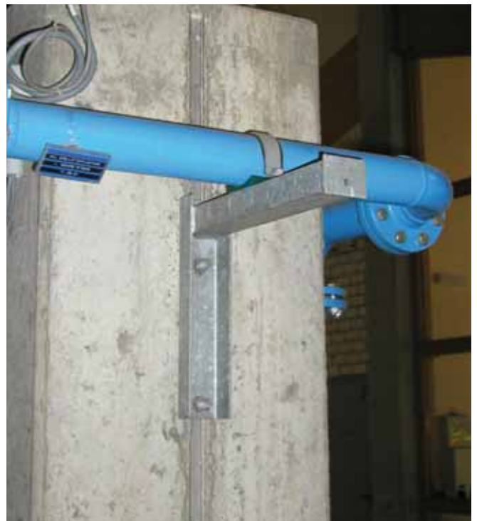
Adjustable pipe support using a cantilever with vertical serrated channel
