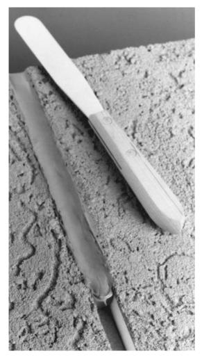
Figure 14.11 Tooling is necessary when sealing edges of irregular surfaces. (Photo courtesy of Polymeric Systems Inc.)
