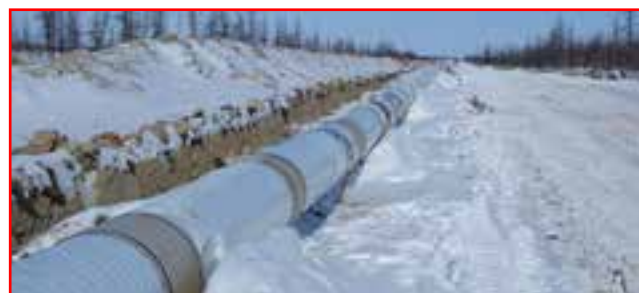
Completed Skin Trace system prior to burying
