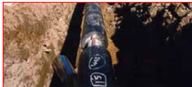
Buried, Pre-insulated Pipe with Longline HTS3F
