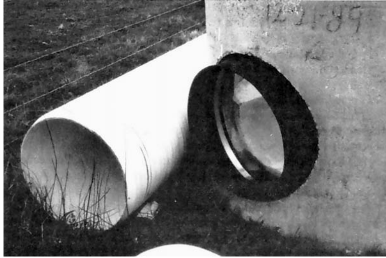
Fig. 12.13 An example of a watertight manhole connection.
