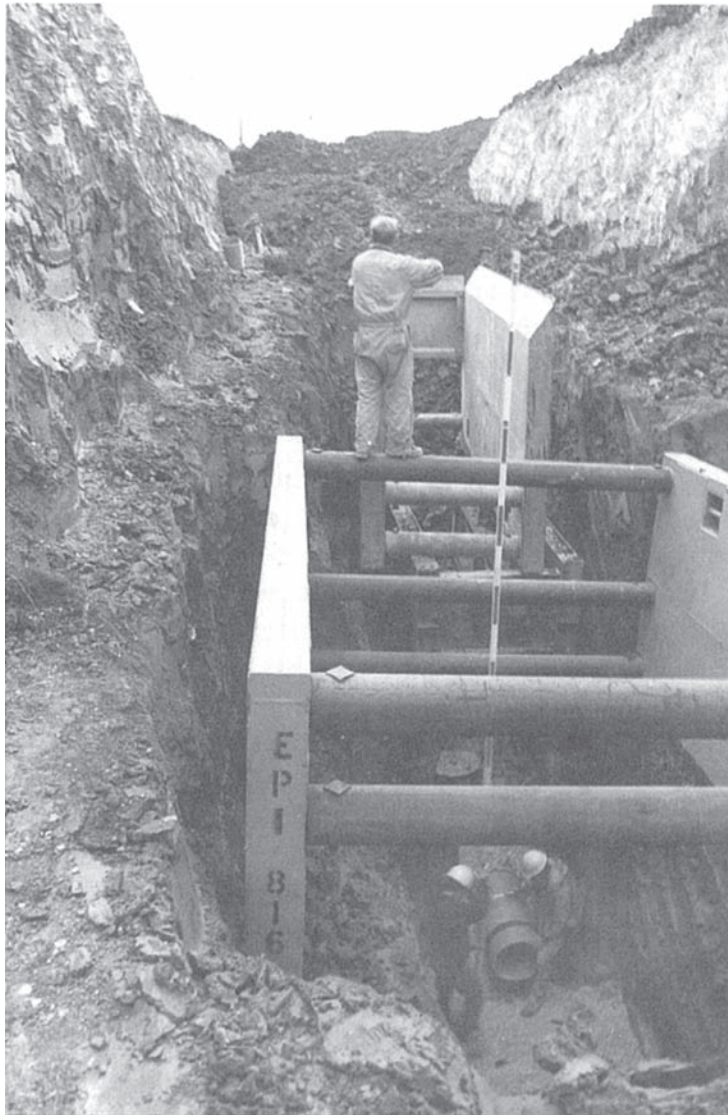
Trench safety is especially important in deep installations.
