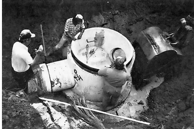
Fig. 12.16 Placing a gasketed pipe joint within 3 ft of each side of the manhole helps to accommodate possible manhole settlement.
