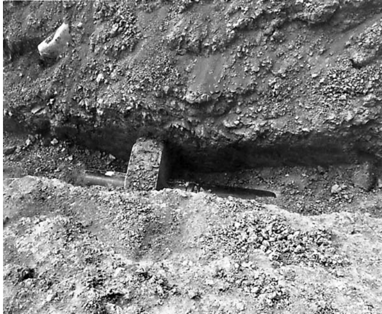
Fig. 12.7 PVC pipe may be anchored on steep slopes.
