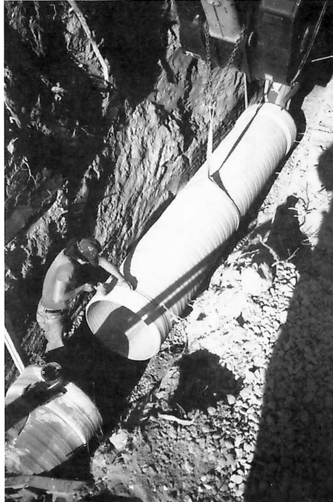
Fig. 12.5 Profile wall pipe installation.
