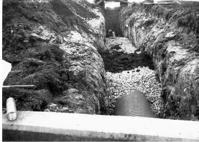
Fig. 12.6 Backfilling with Class I material.
