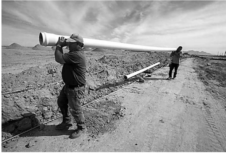
Fig. 10.3 PVC pipe is light enough for manual handling of some sizes.
