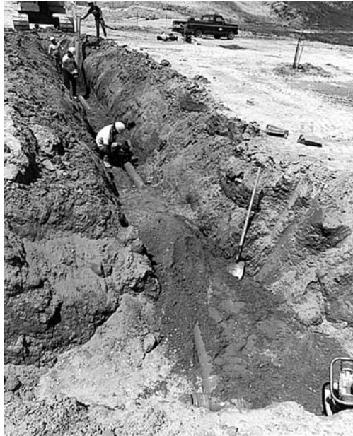
Fig. 8.3 6-in. Class 235 PVC pipe (per AWWA C900 standard) with one length curved in the barrel to required alignment.
