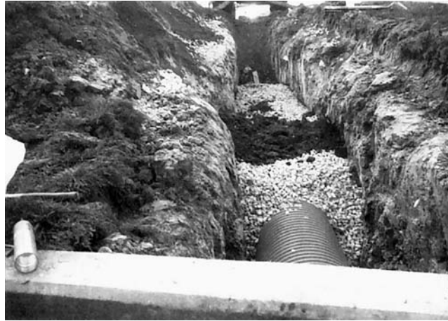
Fig. 12.6 Backfilling with Class I material.
