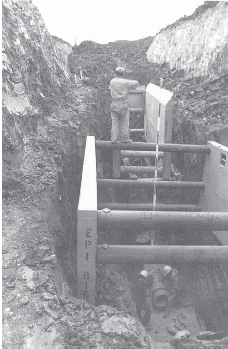
Trench safety is especially important in deep installations.
