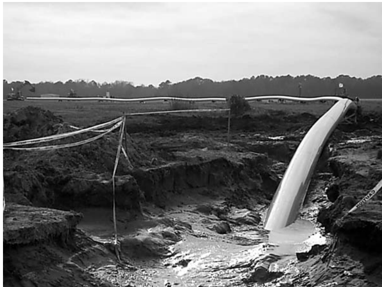
Fig. 8.1 24-in. DR 18 fused PVC pipe longitudinally deflected horizontally and vertically during trenchless pull-in.
