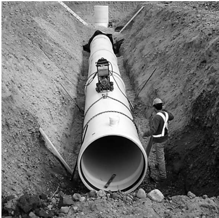
Fig. 10.7 Hydraulic pipe puller.
