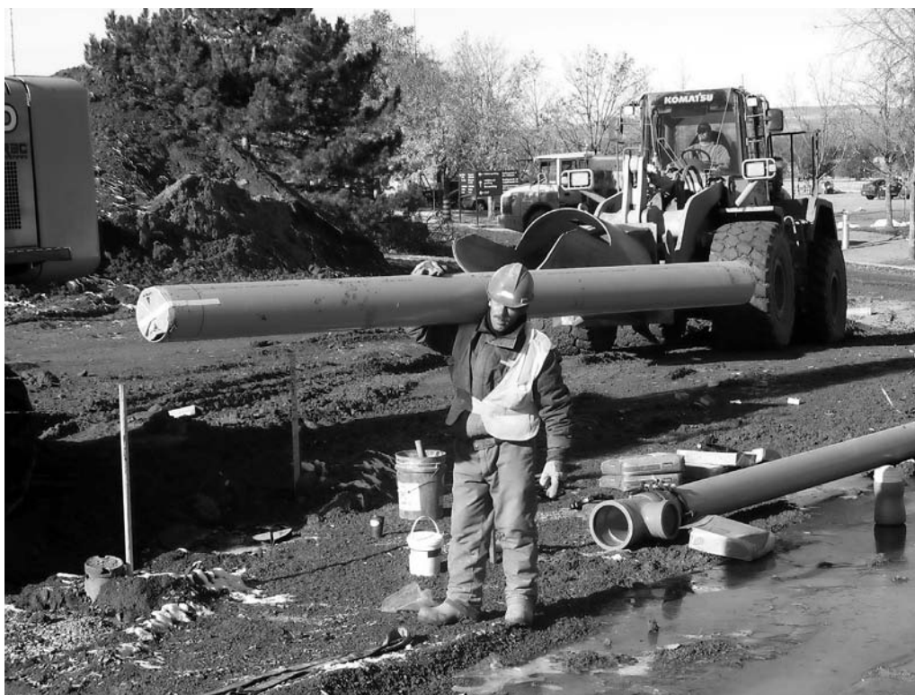
Fig. 14.2 Ightweight PVCO pipe at a job site
