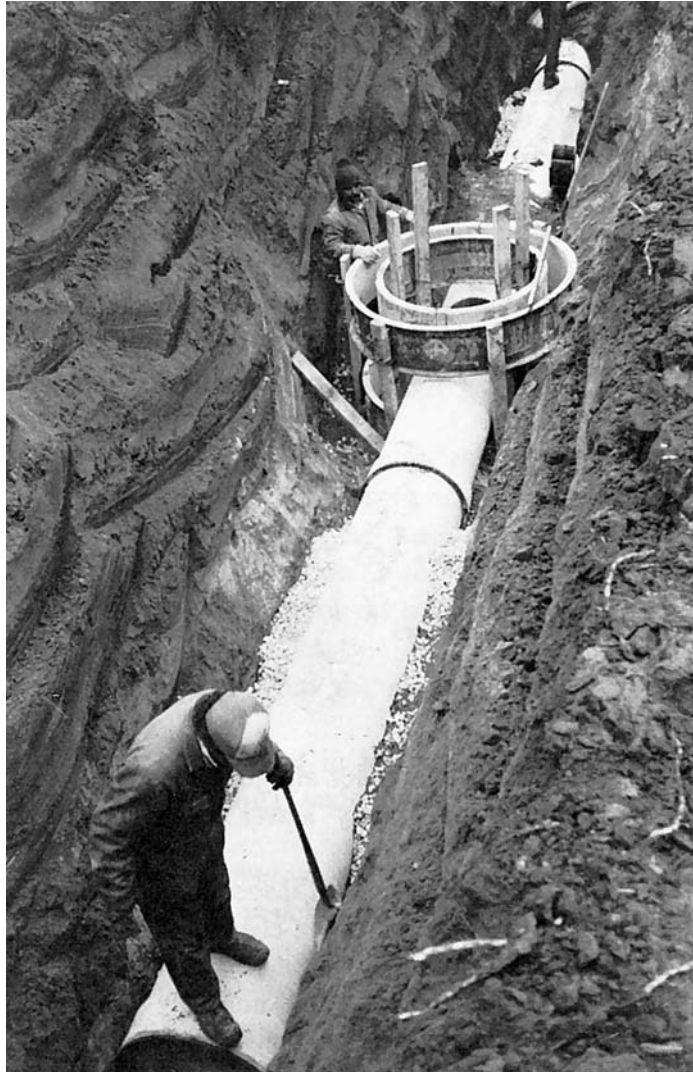
Fig. 12.12 Sewer pipe laid through and beyond manhole location prior to construction of manhole.
