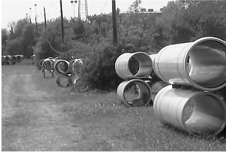
Fig. 10.2 PVC pipe stored on level ground.
