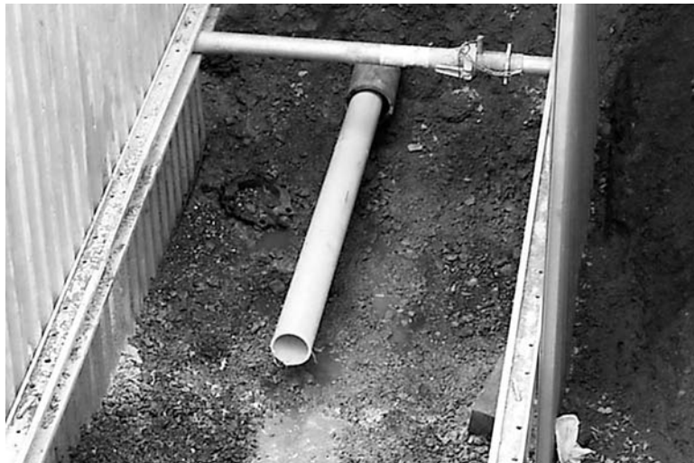
Fig. 13.14 Starting stock inserted into host pipe.
