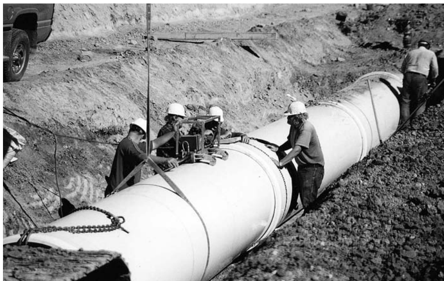
Fig. 1.1 48-inch PVC pipe installation.
