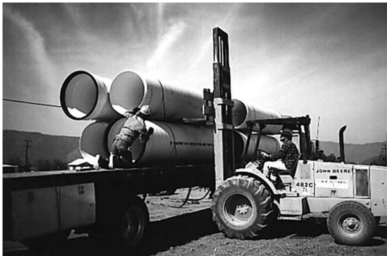
Fig. 10.1 Unloading PVC pipe with a fork truck.
