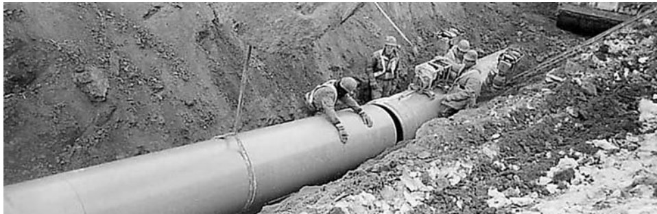
Fig. 10.4 Assembling a pipe joint.
