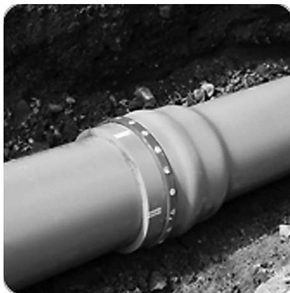
Fig. 13.2 Pin-and groove gasketed joint.
