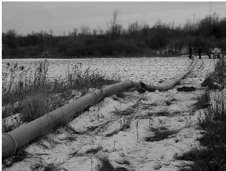
Fig. 13.8 Preassembled PVC pipes.
