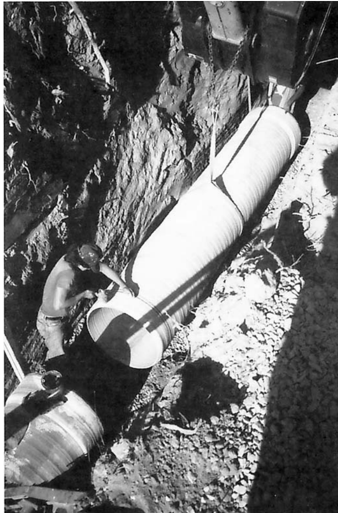
Fig. 12.5 Profile wall pipe installation.
