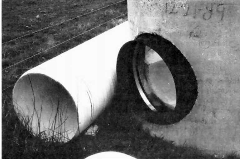
Fig. 12.13 An example of a watertight manhole connection.
