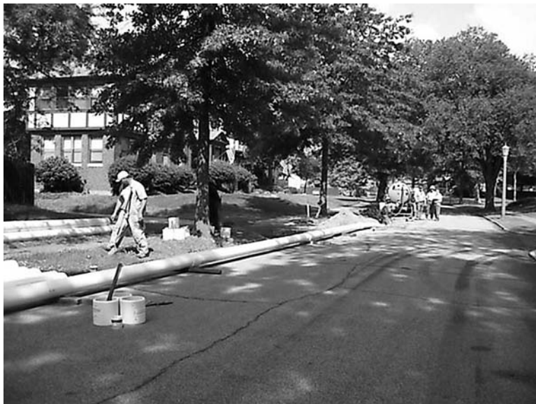
Fig. 13.10 Pipe string during pullback operation.
