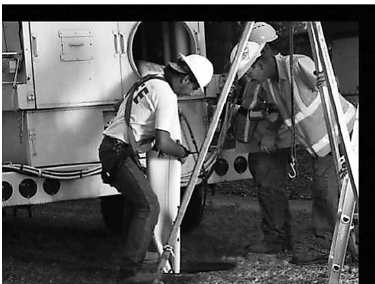
Fig. 13.17 Heated liner being winched into a manhole.
