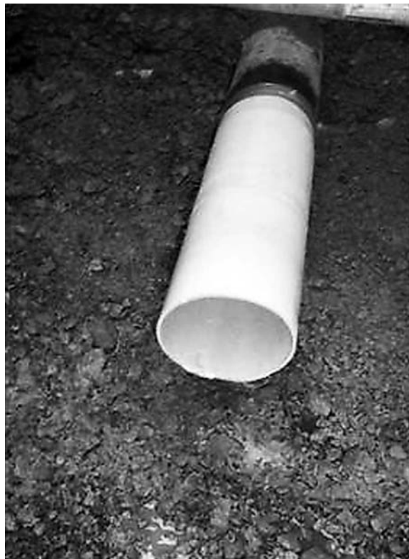
Fig. 13.16 Expanded structural liner with end sized to accept host pipe fittings.
