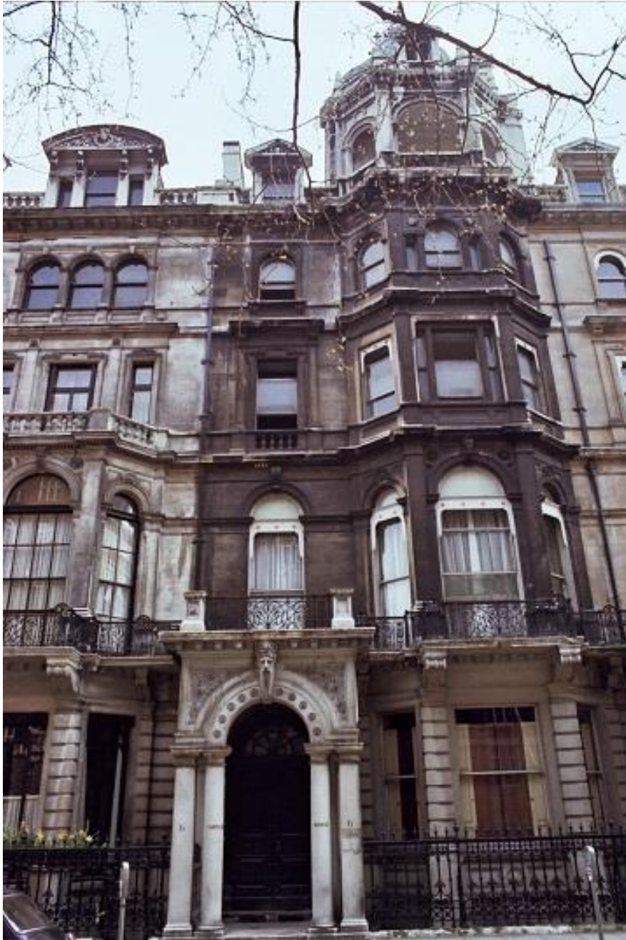
Caroline House before renovation. Photo: Hans Knot
